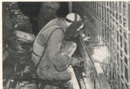
Inner and outer mats are welded at laps (above), joined by brazed leads. Leads also join mats to structural members (below)
