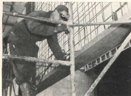
Inner and outer mats are welded at laps (above), joined by brazed leads. Leads also join mats to structural members (below)
