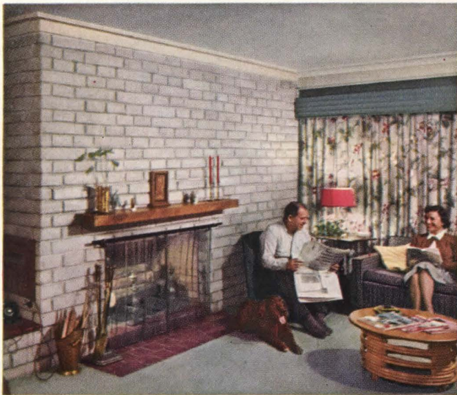
Fireplace of concrete slump block has raked joints for interest
