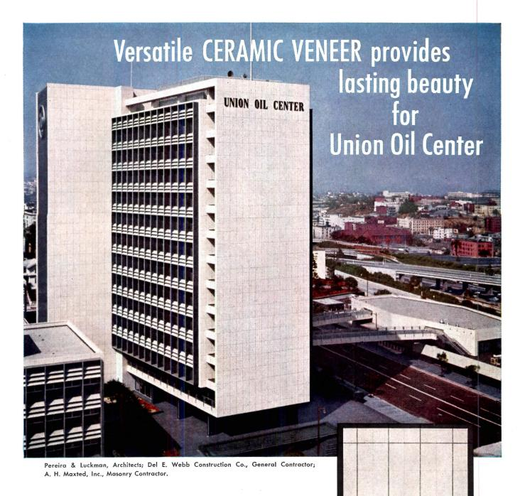
The new Union Oil Center in Los Angeles is distinguished by the effective use of light-grey adhesion type Ceramic Veneer.
