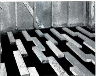
flooring, 12" on centers with ends lapped 4". Staggered pattern helps to provide good nailing surface.
