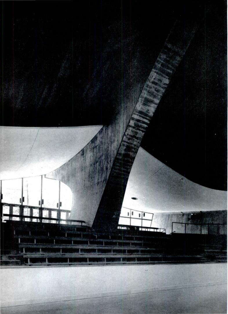
Left: one of two main buttresses of spine at opposite ends of rink's long axis. Plaster ceiling is suspended above seats. Plank roof will be left exposed over rink
