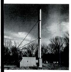
Van-Packer Stack with Hi-Temp Sections handles industrial incinerators with flue gas temperatures up to 2000° F.
