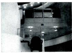
4. View of control room from main floor, circular crane track above, hot end of pool at left
