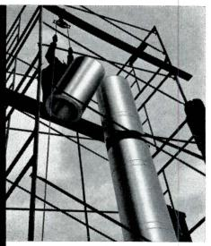
Van-Packer Stack with Standard Sections handles boilers and furnaces efficiently. Can be superimposed or floor supported.
