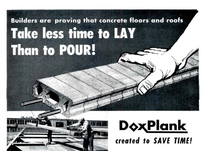
DoxPlank crane-hoisted to Time-Table scheduled position—laid in proper alignment in record time. Provides immediate working deck for following trades.
