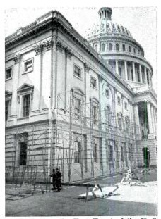
Scaffolding on the East Front of the U.S. Capitol, in preparation for the work of measuring and making casts for reproduction in marble after extension
