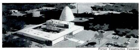
Air view showing garage and pool cooling tower upper left, lab cooling tower in attic oratory rooms. The reactor is a "stock" 5 megawatt pool type using 4.5 kg of Uranium and having walls up to 10 ft thick at the hot end. Air conditioning maintains a slight neg-
