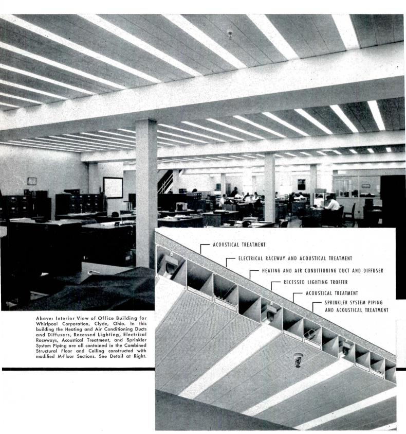
The Cross Section above shows a unique adaptation of M-Floor Construction to provide both the Structural Sub-Floor and Acoustical Ceiling. In this application, Cel-Beams and Channels between Cel-Beams in the M-Floor Sections are ingeniously utilized for several other functional purposes.
