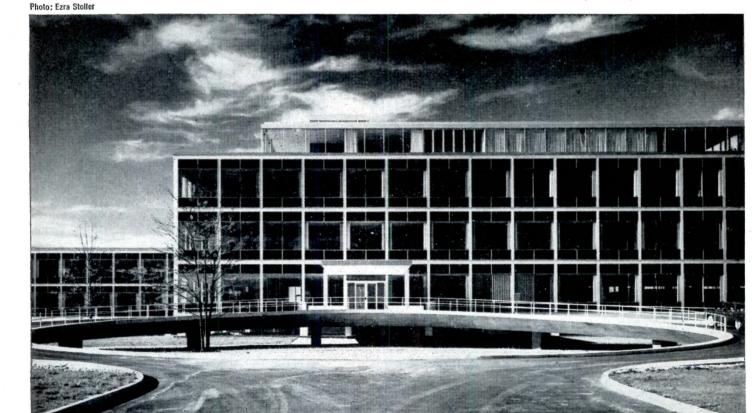
Spandrels are faced with gun metal gray Spandrelite\* backed by a 1" air space and  $1\frac{1}{2}$ " FOAMGLAS insulation. The insulation's unusual strength and rigidity permitted its use without special extra supports. Blocks of cellular glass insulation were also used to fill in the web between the flanges of the steel structural members of the new Connecticut General Headquarters.
