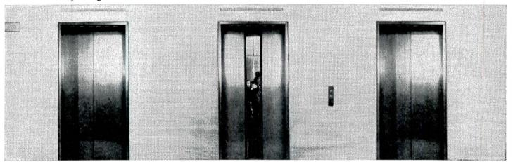
5 "Doors close and elevator will take passengers to their desired floors. No overcrowding. Doors are closed automatically and courteously when the last passenger enters—or when the elevator becomes substantially loaded."
