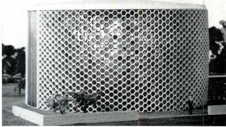
Chapel for Temple Emanuel, East Meadow, L. I., N. Y., has walls of reinforced precast concrete half-hexagonal units, to be laid up in a running bond. This continuous structural skeleton will be filled with colored glasses. Roof structure is still under study. Architects: Davis, Brody & Wisniewski
