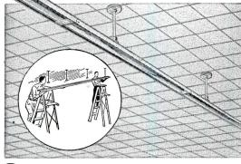
3 Hang the Uni-Race • The rigid Uni-Race is easily lifted and hung in any of several diferent ways. Lengths up to 200' can be hung as a unit if supported every 24' while being raised to mounting position. When the branch-circuit connection is made, the Uni-Race is ready for the fixtures.
