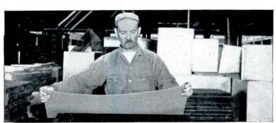
Flexible flashing is quickly adhered to FOAMGLAS blocks to form panel-size units of insulation. Two men easily handled all cutting and assembly operations for the insulated spandrel panels.
