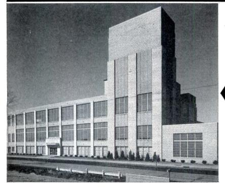
New factory of American Chicle Company, Rockford, Ill. where 14,000 sq. ft. of Coolite Wire glass, Glare Reduced, combines heat absorption with protection.
