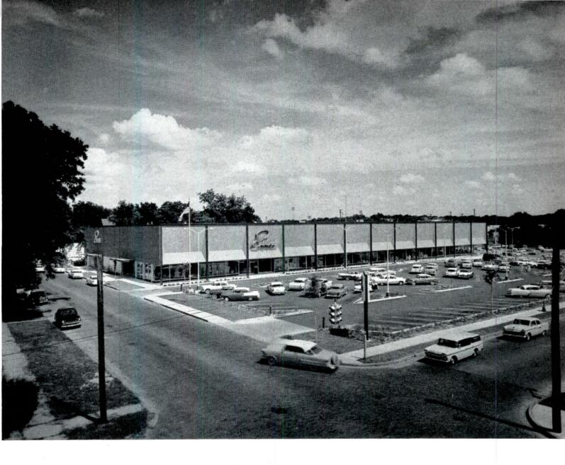
With the exception of the exterior finishes, the construction and materials for the two stores are similar. Both are steel framed with roof slabs of lightweight insulating concrete; interior walls are painted plaster; floors are terrazzo; ceilings are finished with acoustic tile. Both stores are completely air-conditioned, and lighted by a combination of incandescent and fluorescent fixtures
