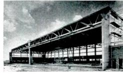
Left: Building while still in progress showing main beam and its relation to seconary beams. Main beam prestressing cables exposed near center column. Below: Completed building, airline administrative offices to the left
