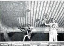
Machine plasterer fills flutes with material. Spot troweling only is required. Finish fireproofing coat is then applied.
