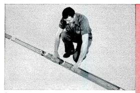
1 Assemble the Uni-Race • The exclusive Gibson Raceway, known as the Uni-Race, can be assembled on the floor in lengths up to 200 feet. The four or eight-foot sections are joined by telescoping couplers which provide a smooth, rigid union of the sections and are fastened with self-tapping screws.
