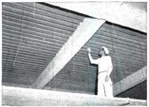
Underside of steel deck prior to application of Zonolite Direct-to-Steel Fireproofing. Oil, dirt removed for strong bond.
