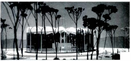
Structure is concrete, formed in place. Exterior columns support beams framing into a central cylinder which shelters the altar and admits light from its ceiling intersection while acting as a column. Shells would be formed on the ground, lifted into place and grouted to each other and the intersection beam
