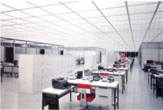
Flexibility of the Reynolds offices is obvious. Partitions can be easily moved to expand or decrease the size of various areas, whereas the Curtis wall-to-wall ceiling of light supplies 75 foot candles of maintained illumination. Curtis grid system is mounted 10 ft. 6 in. above floor level, with lamps spaced 16 in. on center. Hexel Honevite aluminum diffusers complement the decor
