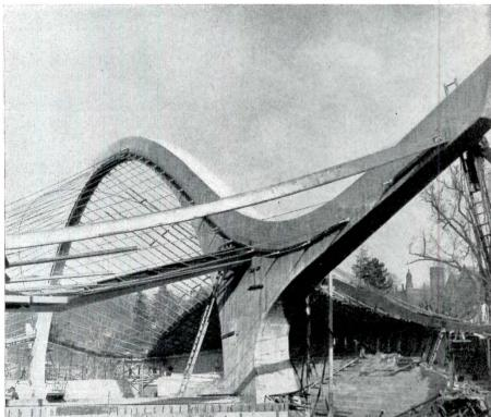
Right: the central supporting spine spans 240 ft as a parabolic arch, then with reverse curvature it cantilevers an additional 40 ft at both ends
