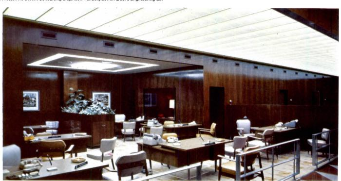
Curtis Strato-Lux provides high levels of glare-free illumination to promote efficiency and serenity. Even with Strato-Lux directly overhead, there are no bright spots, no reflections, in critical viewing areas. Exceptionally low ceiling brightness is achieved through use of #6025 Holophane acrylic plastic Controlens.
