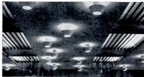
CAFETERIA for Middleville Road High School, Northport, N.Y., features dropped ceiling panels highlighted by a decorative random pattern of gaily colored "spots" adapted from a standard fixture. Fluorescent tubes mounted atop the panel edges supplement the downlighting by casting an even glow over the bright orange-painted cellular decking; above
