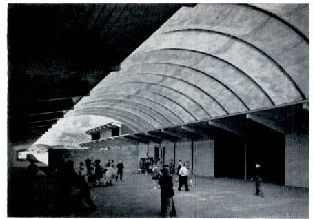
NEW USE OF EXISTING MATE-RIALS: an available plastic product has been skillfully adapted to roof several playsheds between buildings in the Phantom Lake Elementry School, Bellevue, Washington. Installed cost was substantially less than usual roof. Naramore, Bain, Brady, and Johanson, Architects
