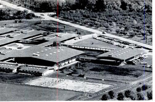
MODULAR COORDINATION: Miramonte High School in California (left), is the first consructed example of the use of Ernest J. Kump's Basic Space Module. This is based on the economic advantage of repetitive components: whole buildings of identical structural, mechanical, and electrical design are repeated many times in a large school
