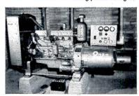
**50KW Onan Model 50KA-4R8,** installed adjacent to the boiler room at the Kenny Institute. Engine operates on natural gas,
