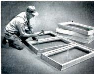
Easy to install. Units are factory assembled, sash hung and weatherstripped. Designed for economical joining into a variety of groupings to fill almost any opening.
