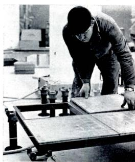
Aluminum Floating Floor plates are set in module frame, covered with standard flooring
