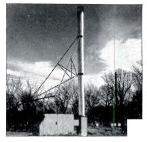
Van-Packer Hi-Temp Stack handles incinerators with flue gas temperatures up to 2000° F. without corroding.
