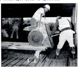
CONCRETING completes the system. Cofar permits wide spans, saves framing, permits earlier occupancy. In a 2-hour UL fire test, Cofar was the first electrified cellular floor system (with header ducts and junction boxes in place) to earn a fire-retardant rating. Optional preset inserts in E/R units eliminate costly concrete drilling. Install floor fittings after building is completed.
