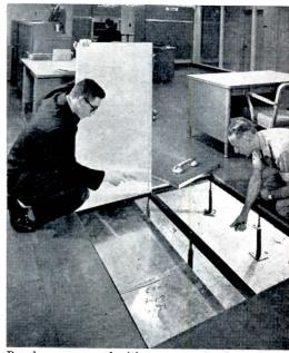
Panels are removed with vacuum-grip, floor leveled by adjusting pedestal height
