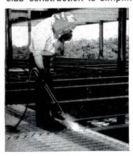
WELDING Cofar and E/R units to framing provides an immediate, strong, safe work platform. No forms to build! Trades move in, days sooner! Wires pulled through E/R raceways can be brought to desks and business machines wherever they are located.
