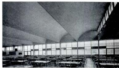
LONG CYLINDRICAL SHELL: Sawtooth arrangement over dining hall at Toyoda Factory, Irolo, Mexico; span 62 ft. With Masso Watanabe, Architect
