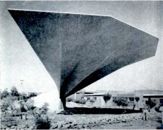
HYPERBOLIC PARABOLOID (Non-vertical axes): Bandshell, Santa Fe, Mexico, D.F. Six h. ps coupled at base to form 40 ft cantilever. Upper edges in tension, lower common edges forming groins in compression. With Mario Pani, Architect.
