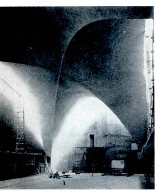
IYPERBOLIC PARABOLOID (Arbitrary curved boundary): Mexican Stock Exchange, Mexico, D.F. Groined vault on a ectangular plan. Edges are inclined for daylighting. Span 85 y 50 ft. With Enrique de la Mora, Architect.
