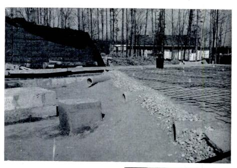
Above: Cross-sectional view of typical intermediate pier slab systems shows (top to bottom) welded wire fabric, plastic vapor barrier, six inches of gravel, floor ducts and uncompacted backfill. A 4 in. reinforced slab will transmit loads to foundation edge walls and intermediate piers.
