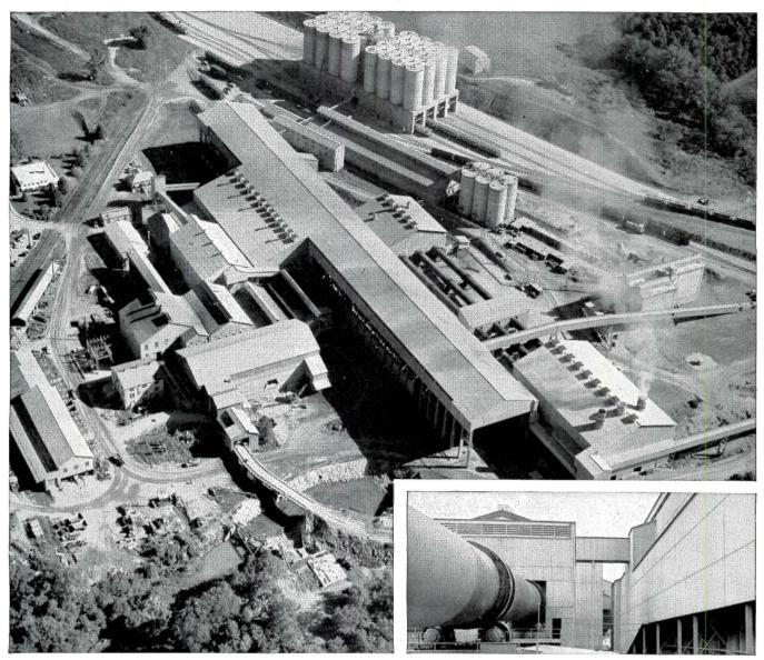
100 acres of "K&M" Heavyweight Corrugated Asbestos went into the expansion of the Union Bridge, Md. plant of Lehigh Portland Cement Co., Allentown, Pa. Pipe-like objects at top center are kilns with a 3,000,000 barrel annual capacity.
