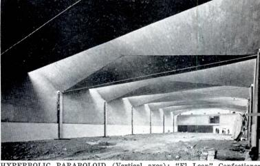
HYPERBOLIC PARABOLOID (Vertical axes): "El Leon" Confectioner; Factory, Mexico, D.F. "Half-umbrellas" spanning 66 ft in sawtooth. Ties are necessary to take lateral thrusts
