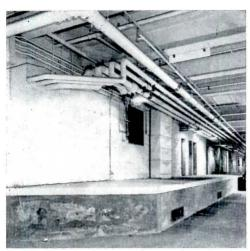
Looking north along truck tunnel at heating plant loading dock; shows hot and cold mains along ceiling.
