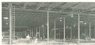
Under Roof — V-LOK steel framing provides the ideal support for Macomber steel deck roofing. Workers were able to proceed with interior construction without delay.
