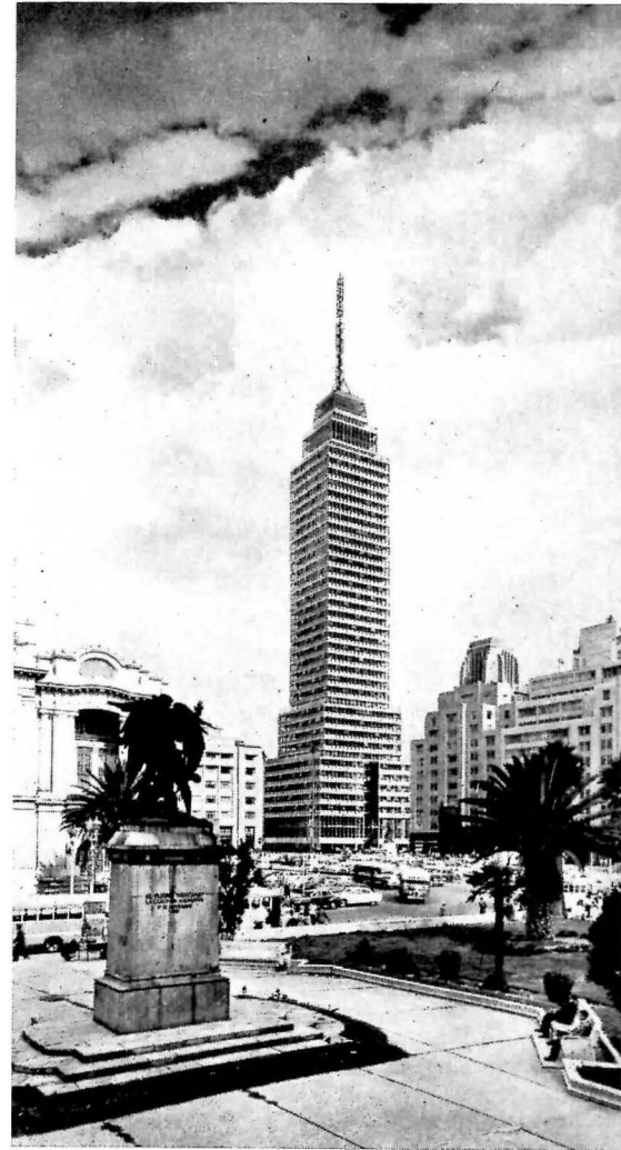
Recent quakes were "proof of the pudding" for aseismic design of Mexico City's lone skyscraper, the 43-story Tower Latino Americana (above)
