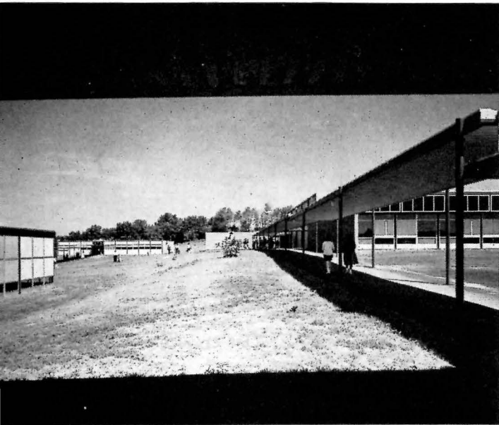
West through center of campus; cafeteria at right
