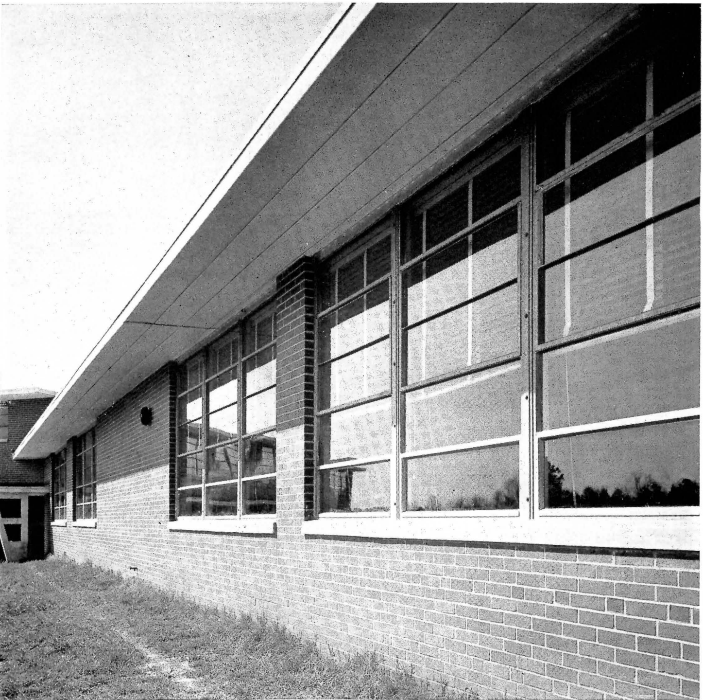
Riverside Elementary & High School , Pendleton, South Carolina, an outstanding example of modern, split-level school design. Contains 38,360 square feet. Capacity: 500 students. 170 Fenestra Intermediate Steel Windows, with their slim, steel members, contribute to the building's architectural beauty, give classrooms better daylighting and ventilation. Architect: John M. Lambert, Jr., A.I.A., Anderson, S. C. Contractor: Triangle Construction Co., Greenville, S. C.
