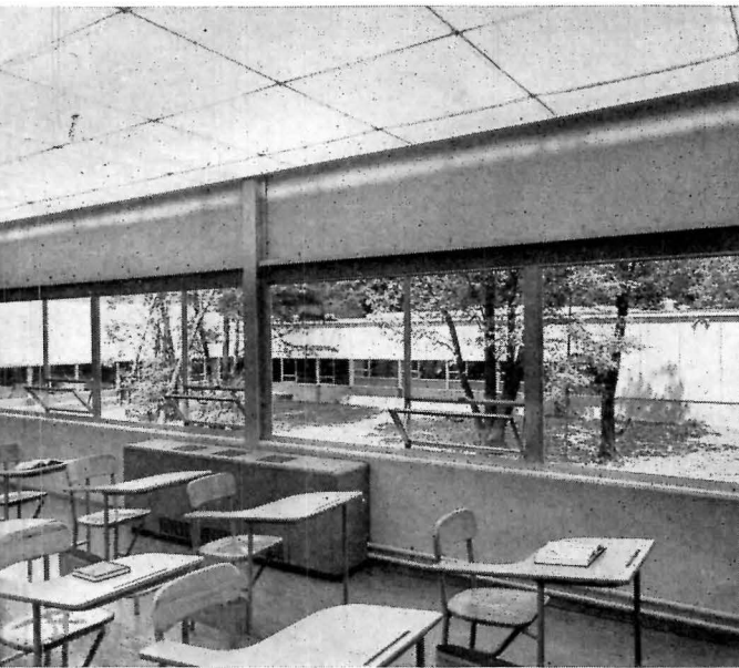
Typical classroom overlooks courtyard to downhill wing
