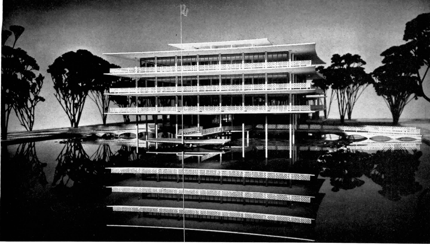
BANGKOK, THAILAND; Embassy Office Building; John Carl Warnecke, Architect. Water in the "klongs," reflecting colorful local architecture, plus heavy rainfall conditions, inspired a delicate, lacy building with wide protective balconies, reflected in a miniature lake
