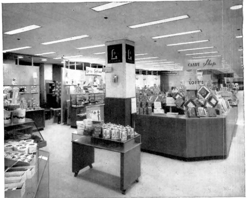
Grinnell Ceiling Sprinklers, which extend but a scant inch and a quarter from the ceiling, provide all but invisible fire protection in attractive display areas, foyers, and executive offices.
