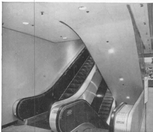
Supplementing Grinnell Ceiling Sprinklers at escalator stairwells is a special Grinnell Water Curtain System, which operates to keep smoke and hot gases from entering open floor areas.
