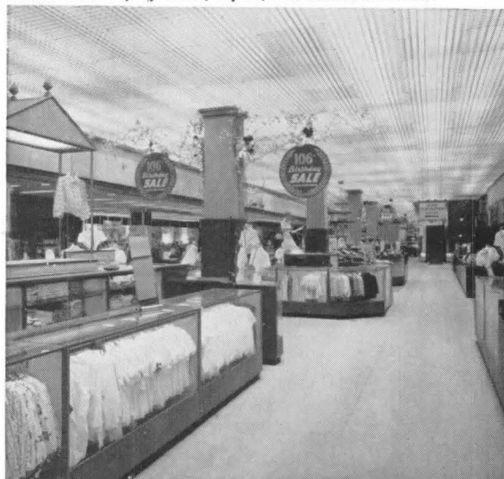
Above this modern ceiling design, not readily seen from below, is the Grinnell Sprinkler System, as well as the indirect lighting.
