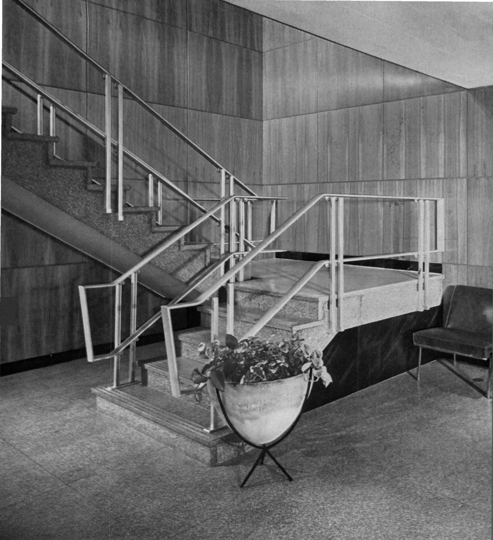
Lobby of Smith-Douglas Co., Inc., building, Norfolk, Virginia. Architectural Woodwork: Elliot and Co. Architect: T. David FitzGibbon.
