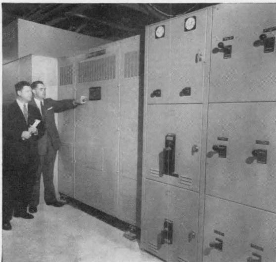
FLEXIBLE double-ended load center unit substation with integrated units furnishes highly dependable power close to load.
