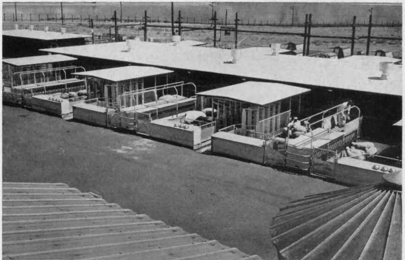
Biological research labs have been built on both "DDD" and "CC" concepts of lab use. Animal housing facilities are sometimes provided in lab building proper, sometimes in separate pens as at Hanford (right). Box labs of special design (left) provide completely controlled environment and mobility of unit for more flexible use of space; care of animal and experiment conditions are simplified
