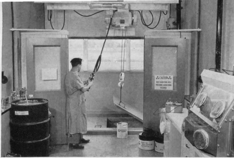
Bulk storage of radioactive material requires controlled conditions to prevent personnel and technical contamination. Heavy shielding—lead, concrete, or water—and isolated location in building are essential. Pool at Battelle Memorial Institute (right) stores lead container under 14 ft of water; crane is needed to handle casks. Pit, before grade, at G-M Lab has 3-ft concrete walls (left)
