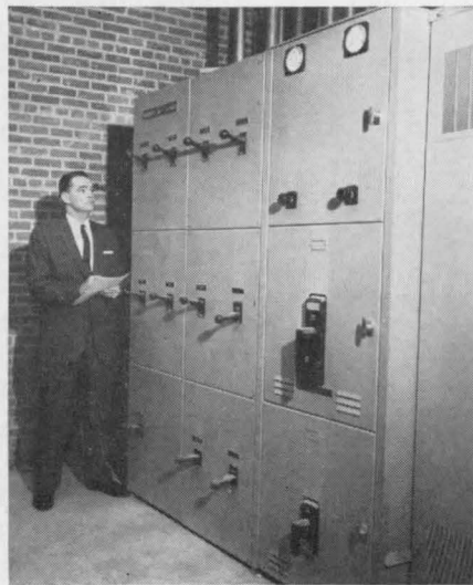
COMPACT low voltage switchgear and distribution switchboard protect low voltage side of "packaged power" system.
