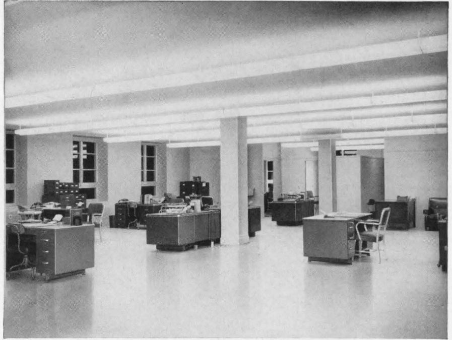
Here's an interior view showing a small part of the installation of Gold Seal Inlaid Linoleum. Actually, about 3½ acres of floor space are covered with this ⅛" burlap-backed "Veltone."
