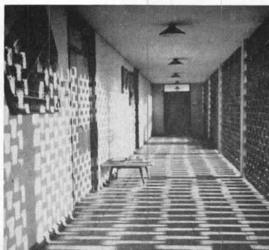
Bottom row, left to right: classroom corridor with sun-screen formed by an open brick grill; looking southwest in garden patio; conference room staff and students in round-table discussion; stairs to library mezzanine; library (mezzanine contains student lounge and space for additional researchers' offices)
