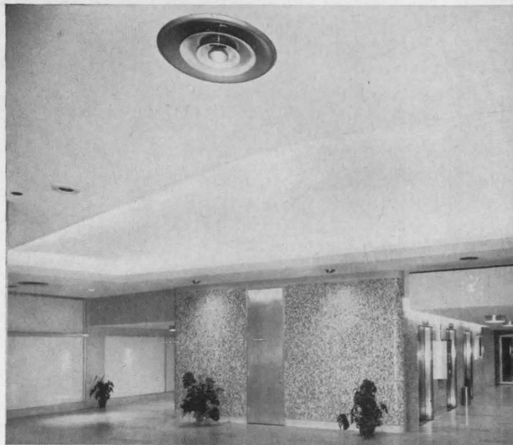
View of lobby showing Anemostat Air Diffusers
