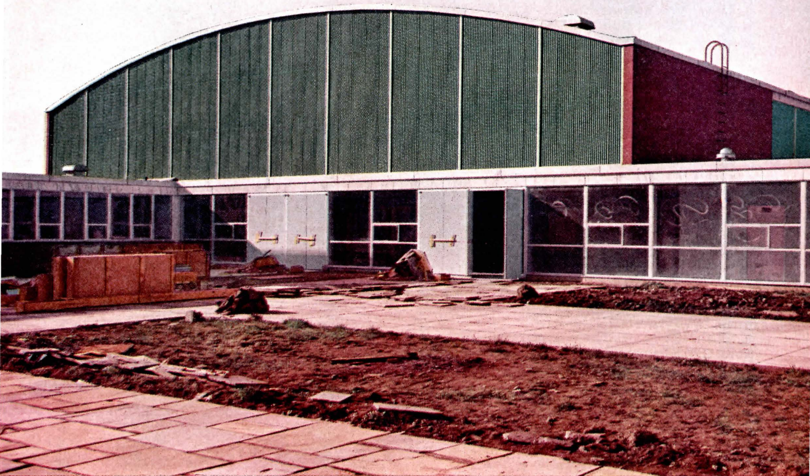
Gymnasium, LaSalle Senior High School, Niagara Falls, N. Y. Architects: Sargent, Webster, Crenshaw & Folley, Syracuse, N. Y. Cannon, Thiele, Betz & Cannon, Niagara Falls, N. Y.
