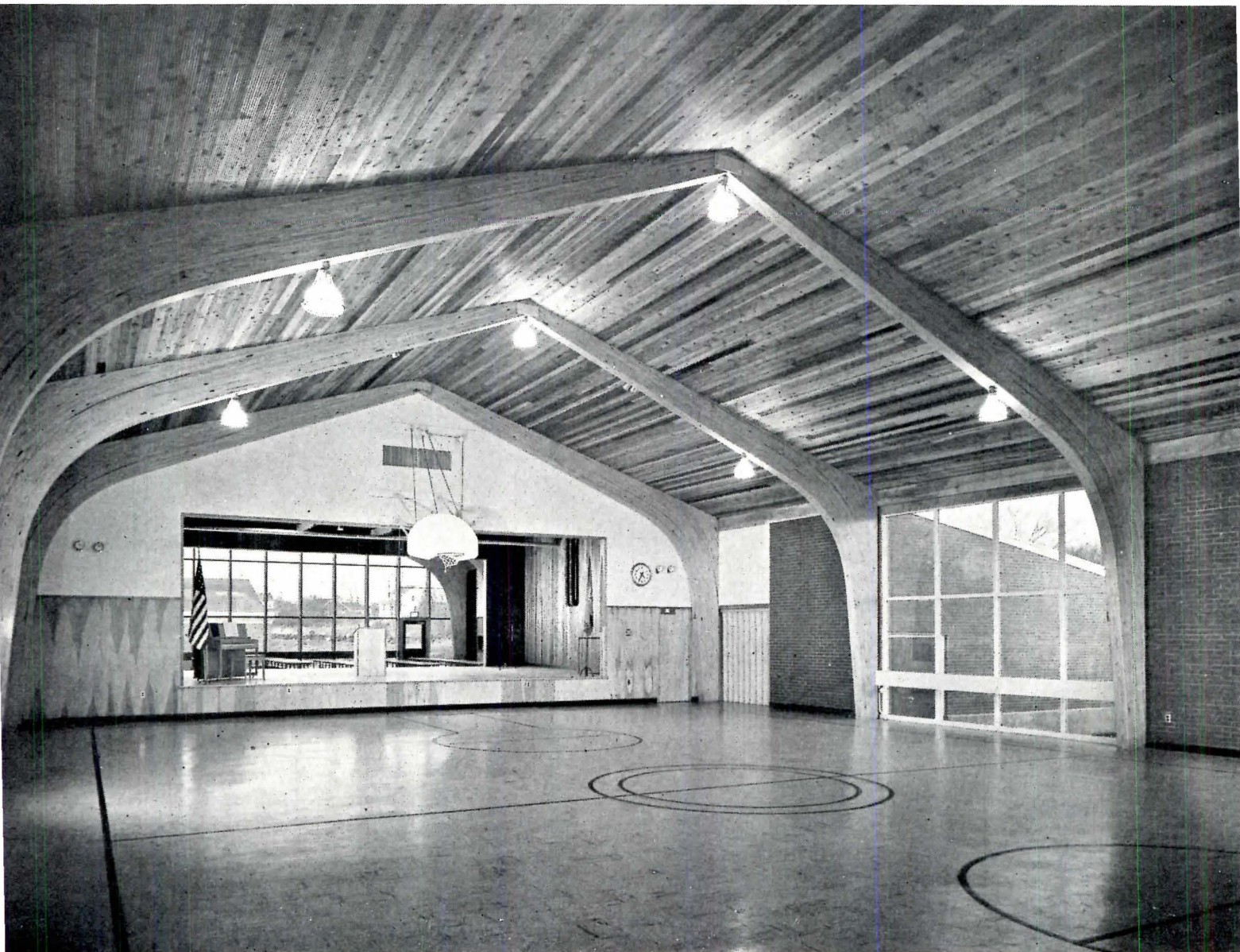
Auditorium-Playroom looking through stage to Cafeteria beyond
