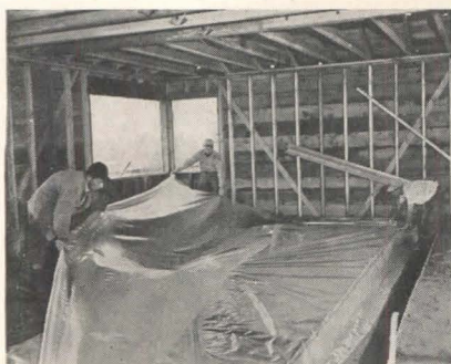
"Some use has been made of polyethylene film as a vapor barrier in walls and ceilings and under poured concrete slabs."
