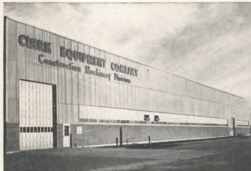
Clark Equipment Company, Construction Machinery Division, Benton Harbor, Mich., 45,630 sq. ft. of 2" Tectum plank for wall insulation.
