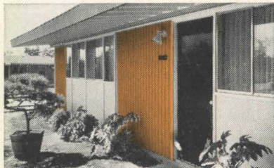
ACCENT flat plywood, masonry and other materials with Texture One-Eleven. Fits new panelized exterior treatments.
