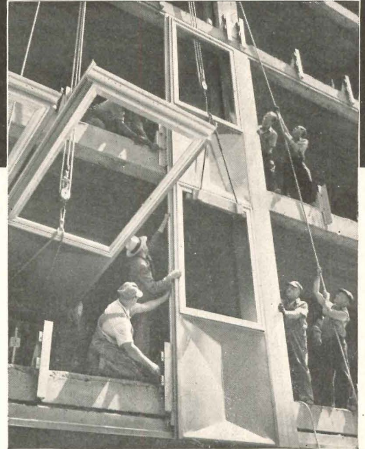
Workmen operating from inside of building, putting aluminum panel into position ready for bolting to steel brackets on framework.
