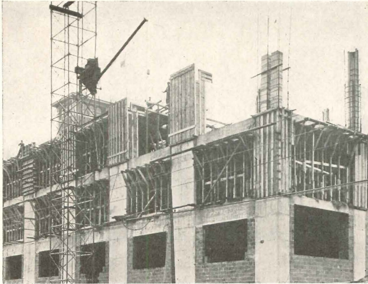
Construction shot shows erection of ventilating columns
