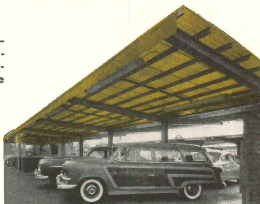
CHEM-O-GLAS UPS SALES — Outdoor showroom of J. A. Eisele Sales, Inc., one of west coast's largest Lincoln-Mercury dealers, showing utilization of CHEM-O-GLAS ribbed structural panels as roofing for structural steel carports.
