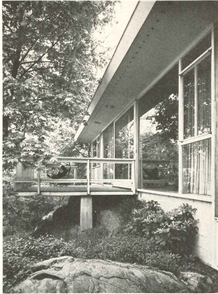
Placement of large glass areas has been carefully studied to center on view, retain privacy
