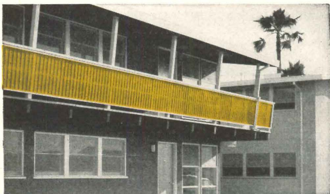
CHEM-O-GLAS (pronounced Kem-O-Glass) is precision molded in 8' lengths, 32 \frac{3}{4} " wide, (32" wide from c/c of outside ribs when overlapped.) Some jobber-dealer territories still open.
