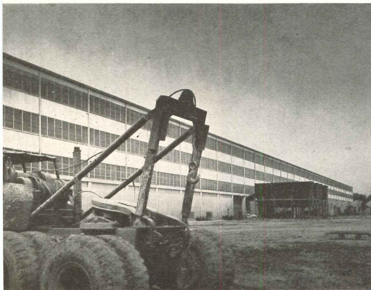
Curtain walls sheath upper portions
