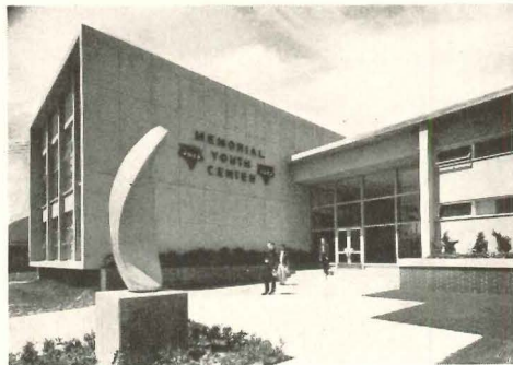
Two more merit award winners: Above: Richmond Memorial Youth Center, Donald L. Hardison, architect. Right: Sunset Community Center, San Francisco, Wurster, Bernardi & Emmons, architects
