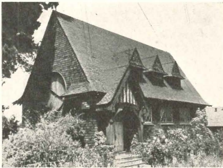
Before and after; Holy Innocents' Episcopal Church, Corte Madera, Crawford & Mann, architects, only remodeling job among winners
