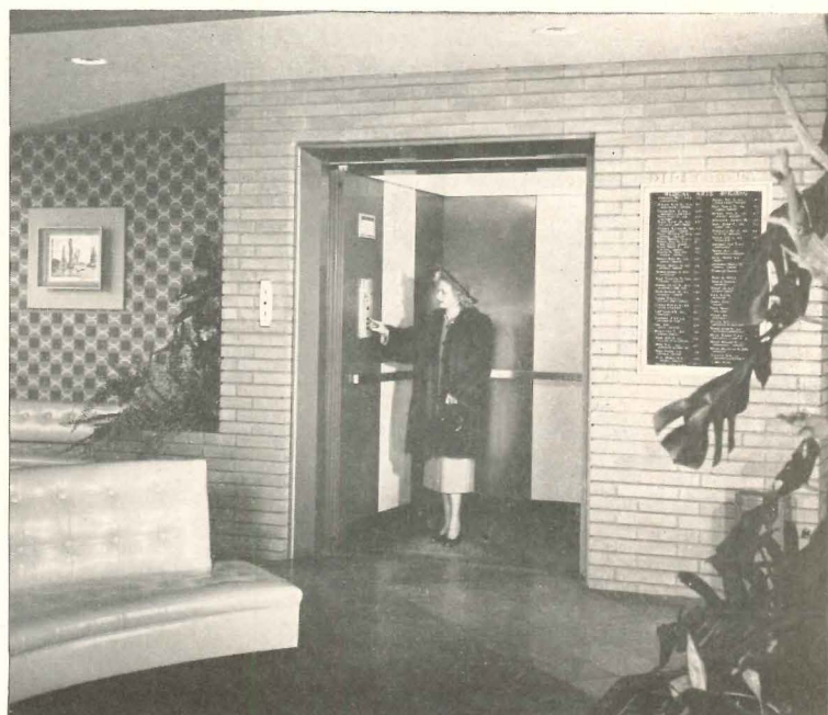
ROTARY OILDRAULIC PASSENGER ELEVATOR SANTA MONICA MEDICAL ARTS BUILDING Santa Monica, California Architect: Weldon J. Fulton, Santa Monica General Contractors: Pozzo Construction Company, Los Angeles Elevator Contractor: Elevator Maintenance Co., Los Angeles
