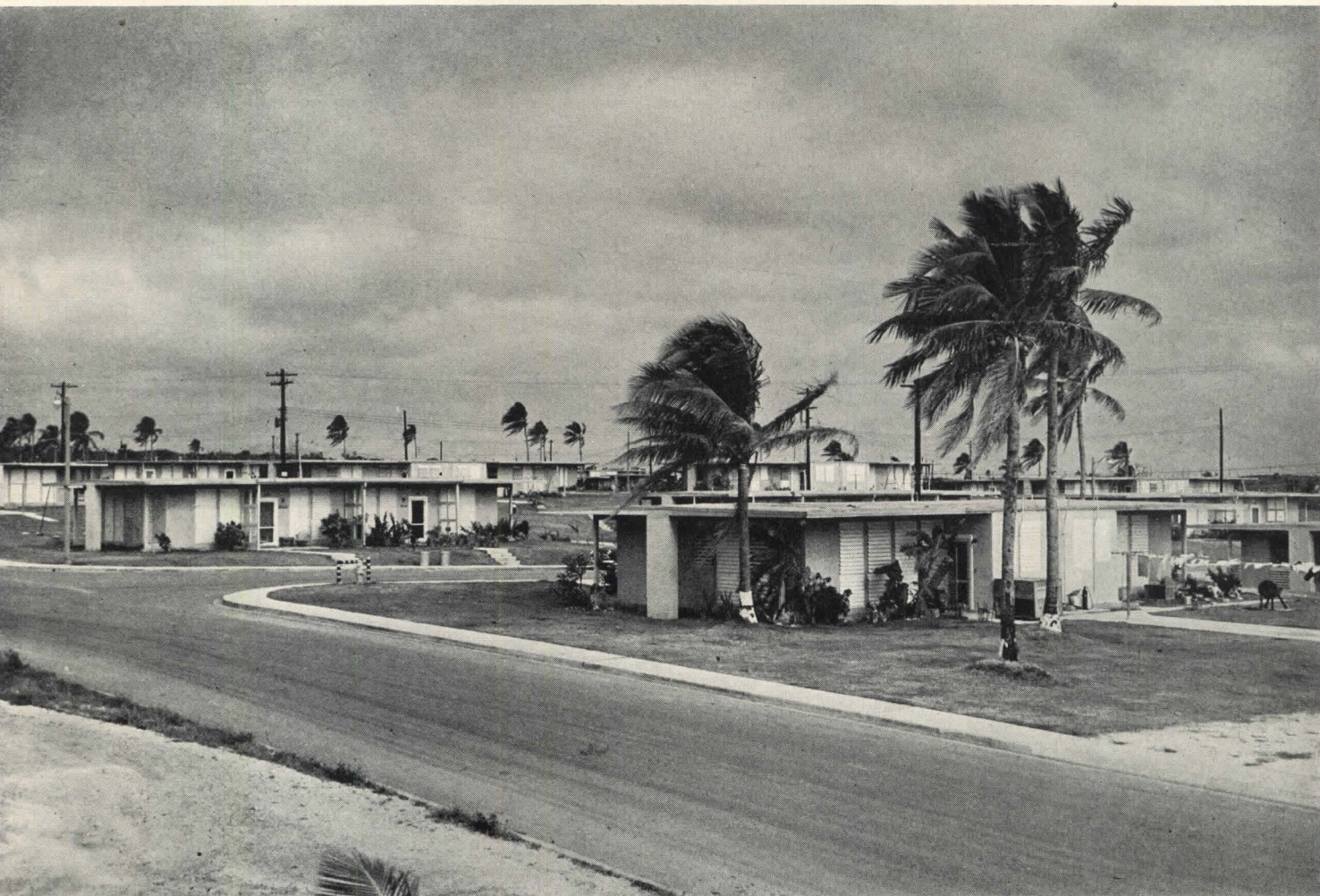
Pacific Island Engineers, Architects
