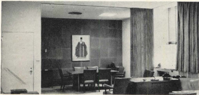
Attractive, modern offices of Henry Sears & Co., New York. Note arrangement of ceiling air diffusers of this central-station air conditioning system.
