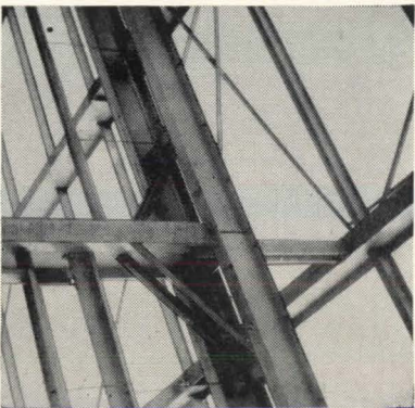
Fig. 1—Simpler Details Method for attaching crane girders to beam columns. Small stub column welded to top of W. F. beam supports roof girder construction.
