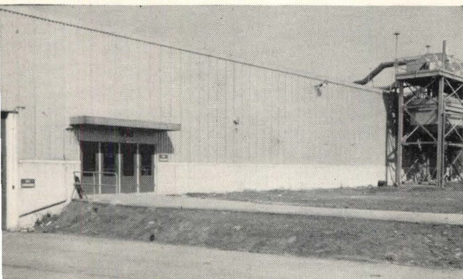
Close-up of the FORMICA plant shows the neat and attractive design formed by continuous Q-Panel fluted texture. Architects have achieved a great variety of design by combining Q-Panels with other materials for decorative effect.
