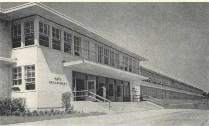
Bureau of Yards and Docks Annex, Washington, D. C. (above)
