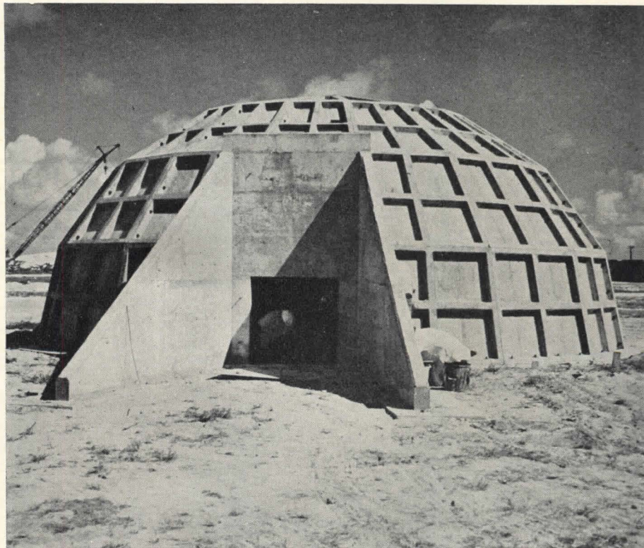
Easily erected panels are of like size in each tier. Units are bolted to precast or poured foundation
