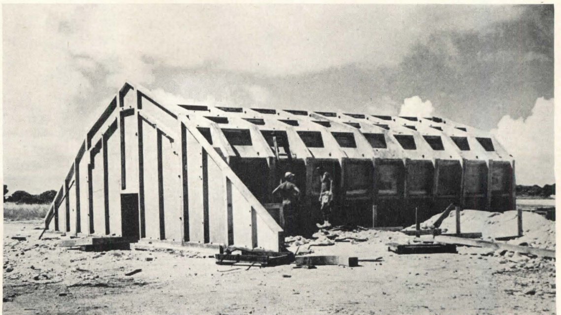
Gable frame shelter provides greater clearance, has deeper ribs to offset less favorable stress pattern
