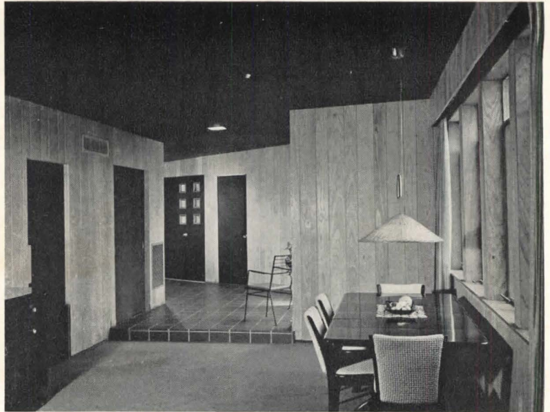
Interior walls of living room (above, left and below) and of entrance hall (above, right) are of natural finish ash. Ceilings are plaster, painted dark brown. Living room floors are wood covered with light green carpet; floors in the entry and on the screen porch are finished with quarry tile. The guest room can be separated from the living areas by a draw curtain
