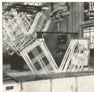
GALVANIZING. Assemblies dip deep into molten zinc, and come up with a thick, smooth, uniform coating. Temperature and timing are automatically controlled with laboratory accuracy.
