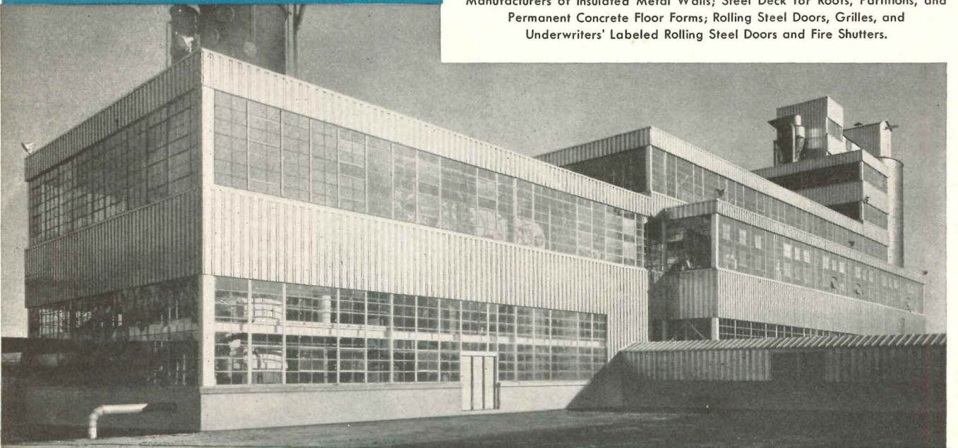
Mahon Aluminum Insulated Metal Walls and Mahon Steel Deck Roofs were employed in the construction of this new plant for Quaker Oats at Omaha, Neb. Verne E. Alden Company, Chicago, Ill., Architects and Engineers. Parsons Construction Co., Omaha, Neb., General Contractors.
