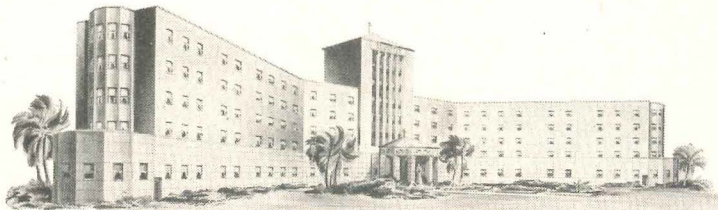
St. Joseph's Hospital. The staff of this new hospital in Phoenix know they can rely on their equipment. Dependability dictated the selection of all materials—including Yale hardware!
