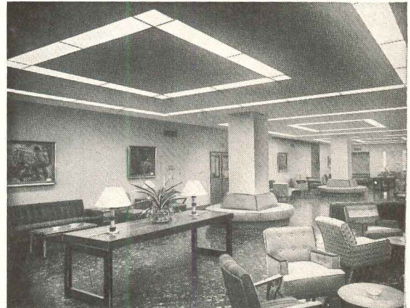
Sylvania Troffers, with Albalite shielding, also provide attractive "pattern" lighting for informal or non-working areas.
