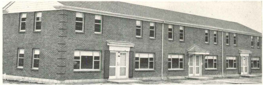
FT. CAMPBELL, KENTUCKY. Wherry Housing Project, Southern Apartments, utilized thousands of Rusco Prime Windows.
