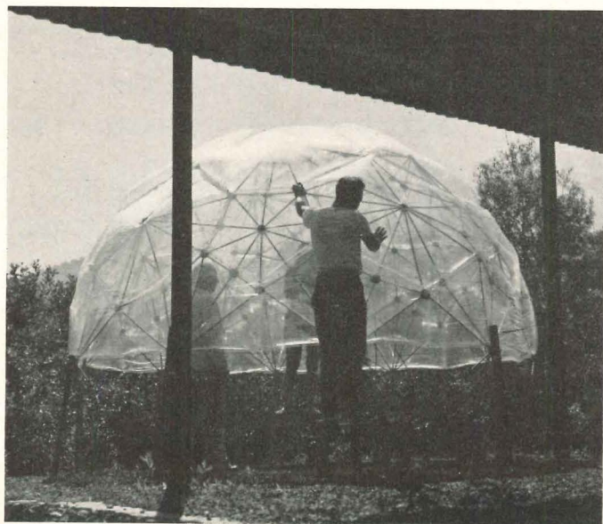
Buckminster Fuller's geodesic dome, shelter design form used by a team of M.I.T. students in planning a theoretical house development on a 275-acre Massachusetts site. The plans were presented for panel discussion at the Jan. 14 housing conference
