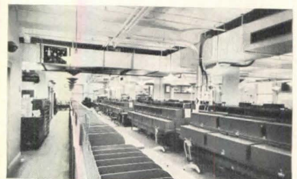
Duct enclosure allows decorative treatment (above). Typical floor duct work (below)
