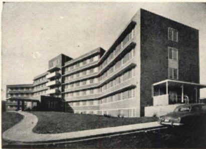
East Tennessee Tuberculosis Hospital, Knoxville, Tenn. Architects and Engineers: Baumann and Baumann; Will W. Griffin and Shi G. Goodwyne, Associates. Heating Contractors: John F. Humphrey Company, Knoxville. Medical Consultants: Dr. R. H. Hutcheson, Commissioner of Public Health and Secretary of the Tennessee TB Commission, and Dr. W. W. Hubbard, Director of Hospital Service for the State of Tennessee.
