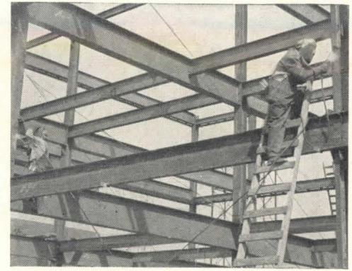
Beam-to-Column Connection used on three story Fenn College Mechanical Engineering Building. Photo shows welders completing column splices.
