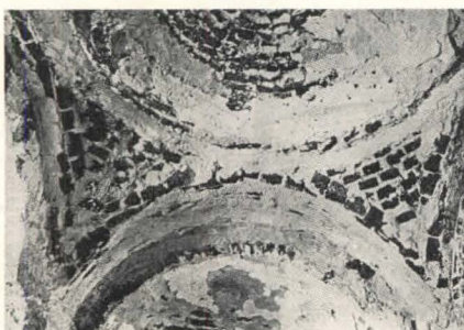
Merging pendentives of brick in St. Menas' tomb, Maryut. 400–410 A.D. Photographs from Roman Sources of Christian Art
