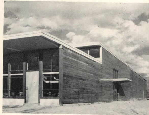
End of classroom wing, multi-purpose room in background. Classroom wing can be extended if future needs require
