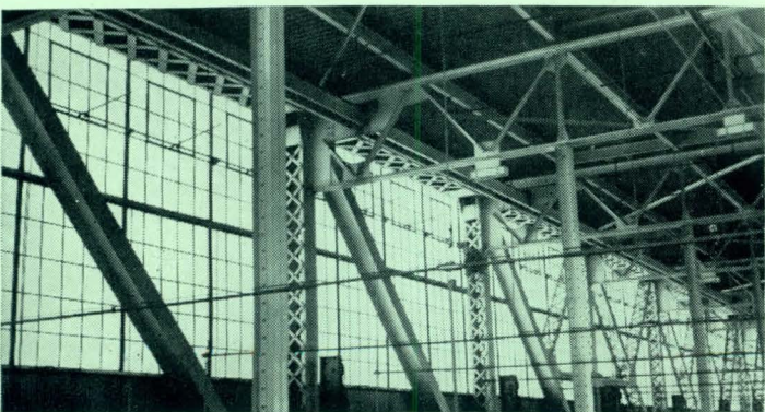
Interior view of Coolite in a southern exposure. Note even distribution of soft, comfortable daylight.
