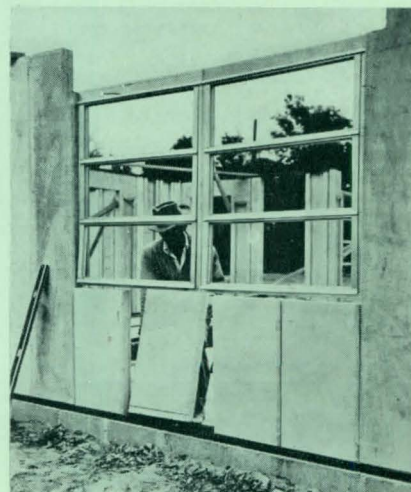
Light-weight structural masonry panels are easily and speedily erected
