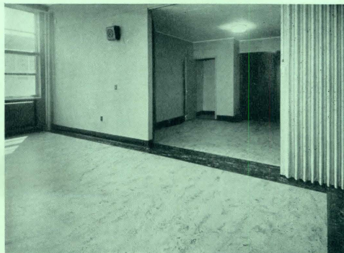
3. Notice the striking decorative effect achieved by the linoleum border in this double room. The room can be adjusted to various uses by closing or opening the flexible partition.
