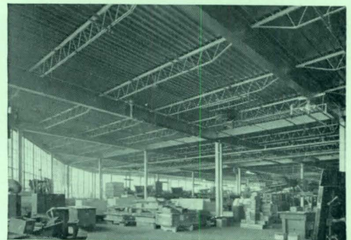
Standard joists span up to 32 feet and Long-span joists up to 64 feet. By using these maximum spans, the number of columns are reduced and more manufacturing area is made available.
