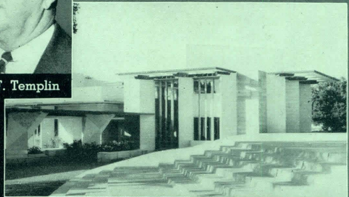
Thoro-seal Protection, Architect, Frank Lloyd Wright. General Contractor, John F. Templin.
