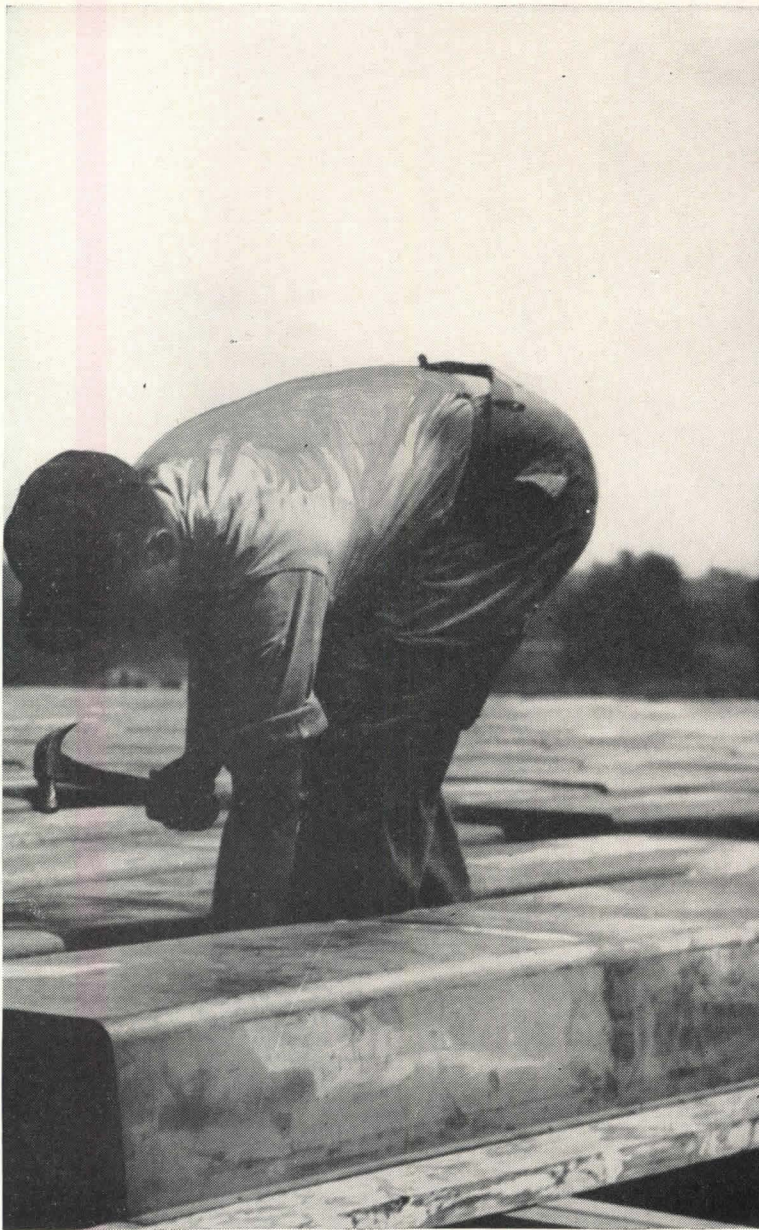
INDUSTRIAL BUILDINGS — Ceco's Meyer steelform method speeds construction: the simple skeleton centering goes up fast; the forms are quickly placed and removed by unskilled labor.
