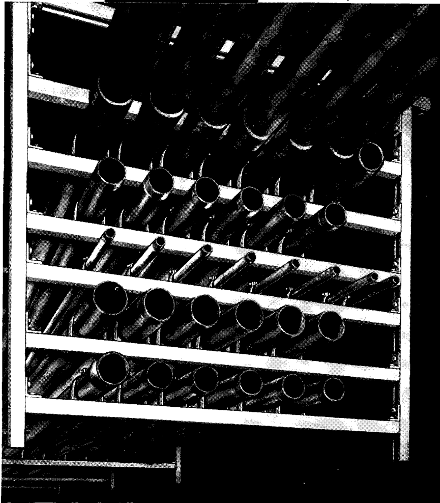
Cross section view of Unistrut-supported heavy conduit run in recent installation at American Sugar Refining Company's Chalmette, Louisiana plant. Note that Unistrut's flexibility makes possible later additions or changes.
