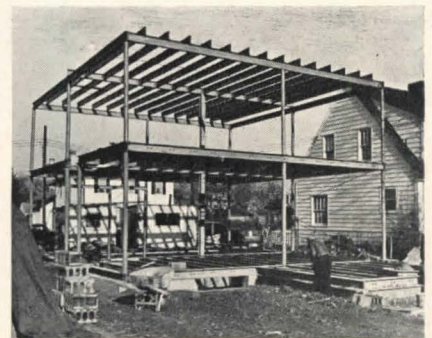
Steel framework for 2½-story house is said to save on labor costs
