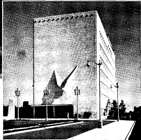
Lounge and exterior, Veterans Memorial Building, Detroit, Mich. Architects and Engineers: Harley, Ellington & Day, Inc., Detroit, Mich. General Contractors: Kuhne-Simmons Co., Inc., Detroit Air Conditioning Contractors: American Refrigerating Co., Detroit
