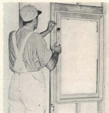
Metal window unit has wood surround for easy installation
