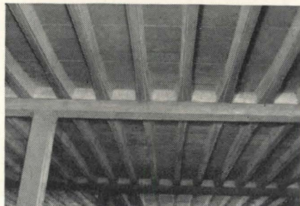
CONCRETE JOISTS eliminate much of the concrete below the neutral axis, saving money, saving material. Suited to buildings with long spans: stores, offices, apartments, hotels.
