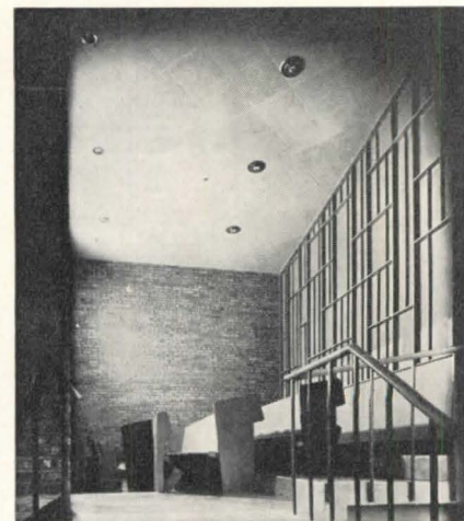
Plastic fabric used to screen pipe-organs gives good tone quality, cleans easily
