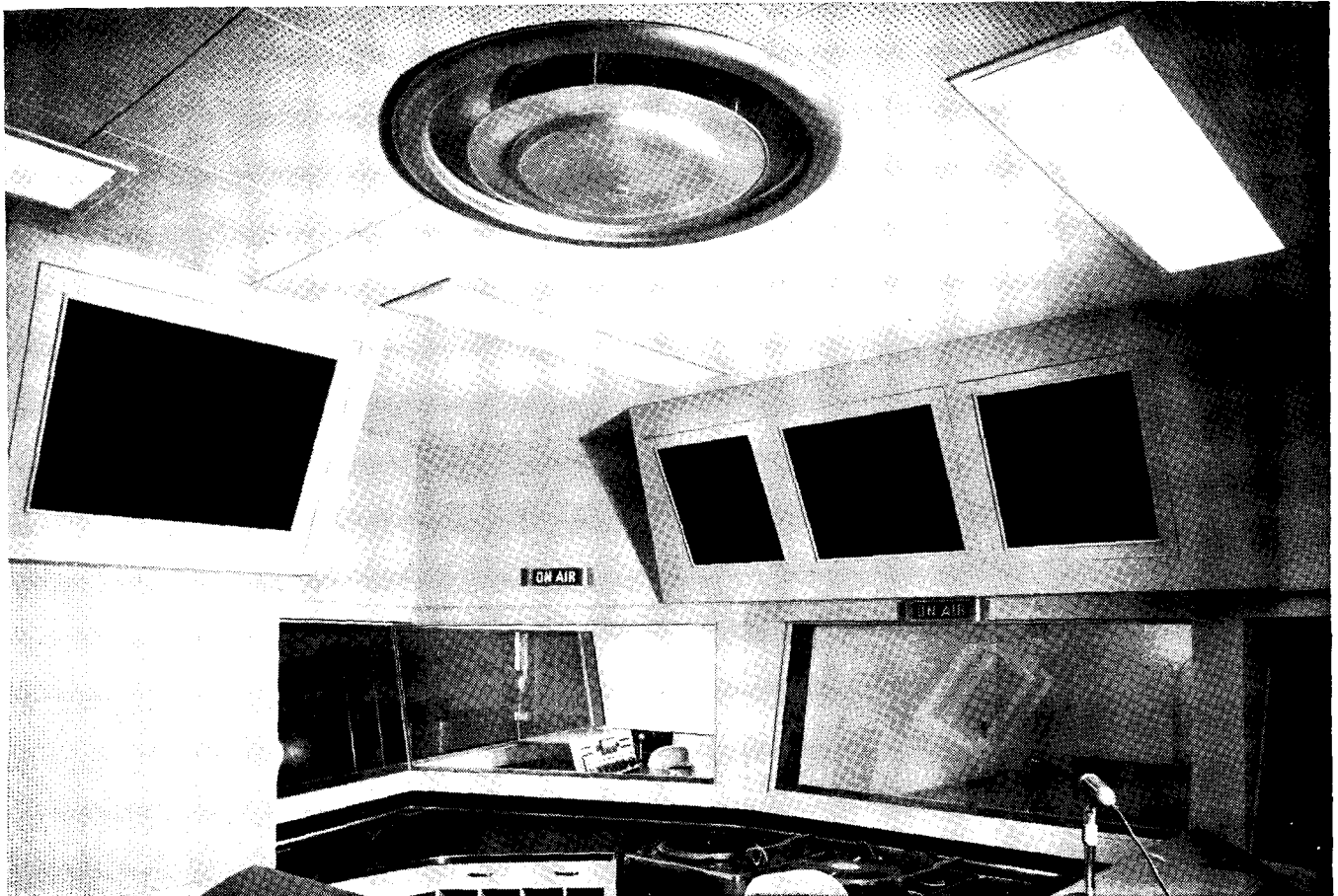
Control Room: Radio Station WFDR, New York, N. Y. Architect: Robin and Vogel, New York, N. Y. Engineer: Fred L. Moesel Associates, New York, N. Y. Mechanical Contractor: The J. M. Fink Co., New York, N. Y.
