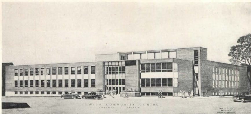
Jewish Community Center in Toronto will be of reinforced concrete construction with brick curtain walls. Besides an auditorium with seating capacity of 600, there will be swimming pool, gymnasium, hand-ball and squash courts and lounges. Page & Steele of Toronto are architects; Kaplan and Sprachman are associate architects
