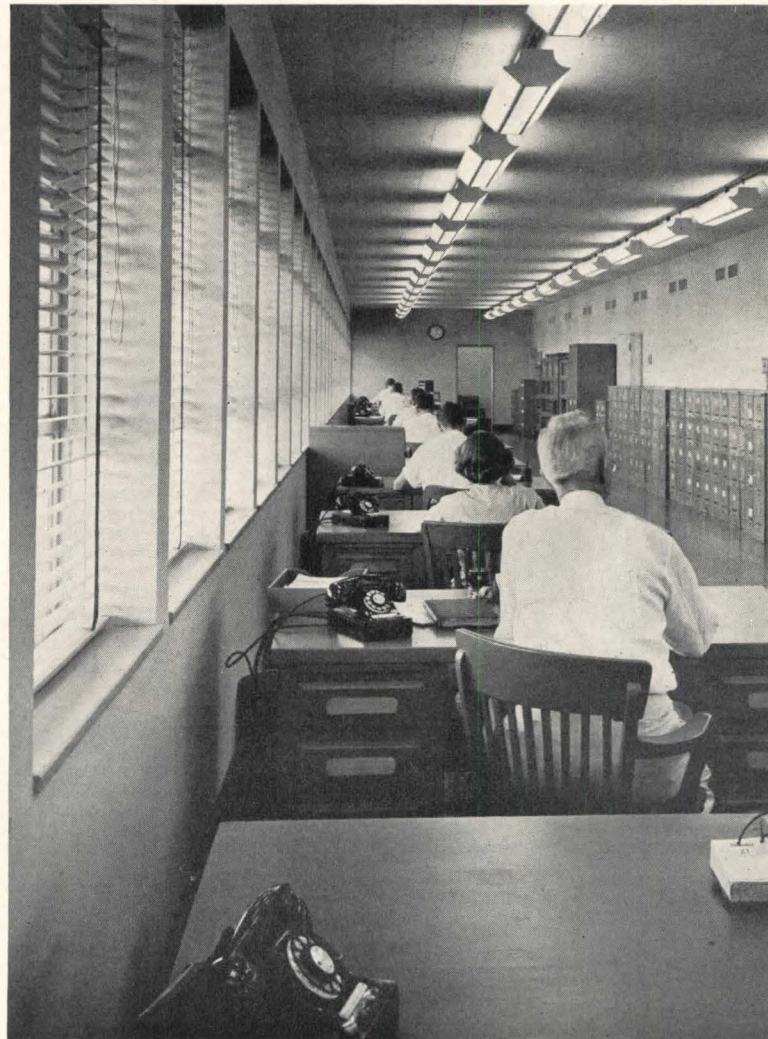
Photograph shows appearance of exterior wall unbroken by projecting columns. Space along outside walls can be used to full effectiveness, whether the area is partitioned or open
