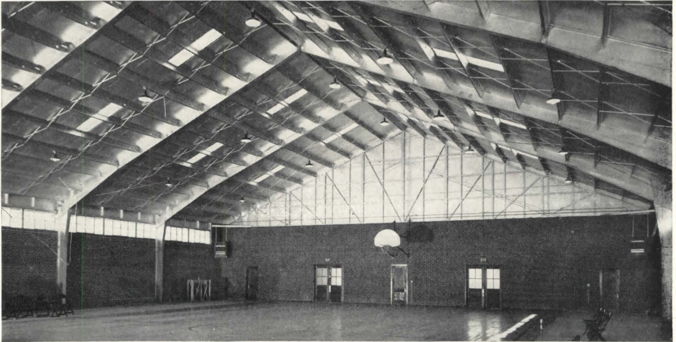
School gymnasium, 82' x 120', at Wright City, Oklahoma. Designed by David R. Graham, Tulsa, Oklahoma. Has clear, unobstructed view from everywhere. Note simple, compact roof construction.
