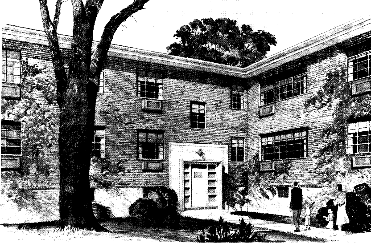
Above: Exterior of Childs Garden Apartments, showing placement of Frigidaire window air conditioners. "It is my conviction," says Robert Meirick, the builder, "that air conditioning is the greatest drawing card in attracting and holding tenants today."
