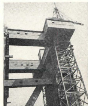
EXCELLENT CORROSION-RESISTANCE. Siding, roofing, gutters and leaders are Monel on the Sherman Creek coal hoist. The 37 years of service that this installation has seen have had little or no effect.
