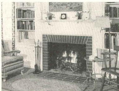
A Colonial Fireplace built around a Heatilator Unit. Warm-air grilles are located in the bookshelf sides.
