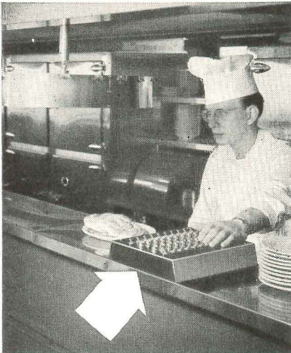
Arrow points to Type RC-20J Single Pole Toggle Switch Control Unit, with Jewel Bull's-Eye Lights and Chime Ringing Buttons operated by chef as order is ready. Waitress turns off switch as she picks up order, clearing lighted numbers from annunciator.
