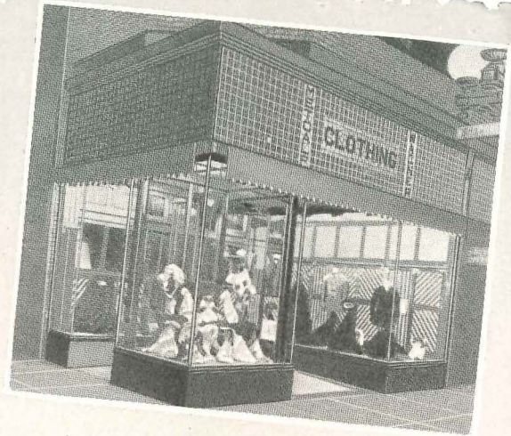
"Modern" BRASCO Installation Vintage of 1917
