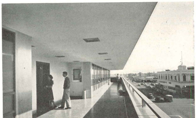
Section and view, exterior corridor, Sill Building, Bakersfield, Calif. (photo: Roger Sturtevant). All services in flush hung ceiling of removable tiles; partitions demountable — an invaluable aid to flexibility
