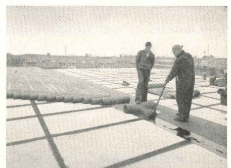
Asphalt roll roofing applied over Cemesto. Pittsfield Township School, Washtenaw, Mich. Architect: C. Nobel. Contractor: DeKenning Const.
