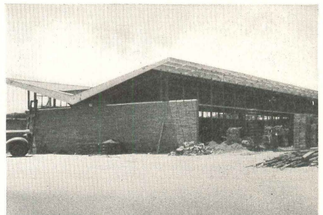
The four buildings comprising the modern design WESTSIDE UNION ELEMENTARY SCHOOL, Lancaster, California, utilize over 10,000 feet of Revere 1/2 inch type L hard temper Copper Water Tube in the radiant panel heating system. Architect: Frank Wynkoop; General Contractor: M. J. Brock & Sons; Heating Contractor: Ray Engineering Co.
