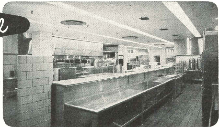
Kitchen of Terrace Plaza Hotel, Cincinnati; Skidmore, Owings and Merrill, Architects
