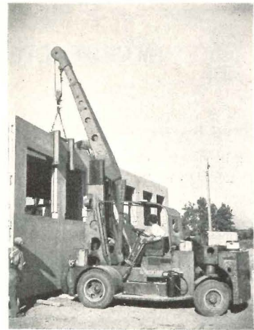
Crane hoists sandwich-type precast panels into place (above). Derrick is used with 16-in. panels of another system (below)
