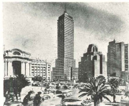
Mexico City's first 40-story building. By La Latino-Americana, Cia. de Seguros Sobre La Vida, S.A., engineering staff
