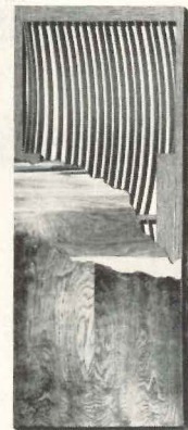
Flush door has arched ribs for support
