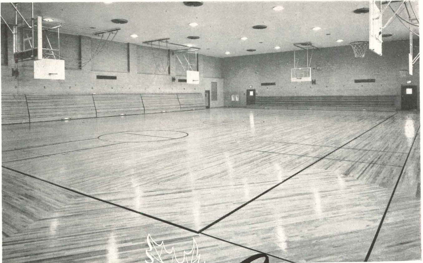
Floor of Northern Hard Maple, 80 x 100 feet, a dual-purpose innovation which combines gymnasium and roller-skating rink, at Archbishop Stepinac High School, White Plains, N. Y.—an interesting development in supervised recreation. Eggers & Higgins, Architects, New York, N. Y.
