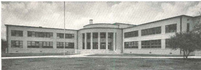
Below: Truscon Donovan Awning-Type Windows used in Ripley Memorial, Houston, Texas.
