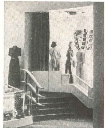
Air conditioning outlet in modern, backless window which extends into the main sales area.
