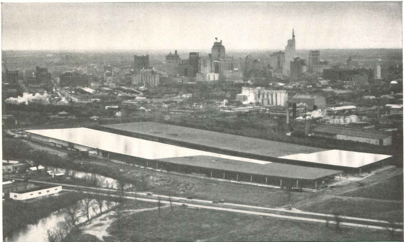
ALFORD REFRIGERATING WAREHOUSES, DALLAS, TEXAS — NOW UNDER CONSTRUCTION, ROOFING CONTRACTOR: LLOYD GRAY, MT. AUBURN ROOFING COMPANY. SPECIFICATIONS FOR THE 23 ACRES OF BUILT-UP ROOF: 2 PLYS OF REYNOLDS .004" EMBOSSED ALUMINUM OVER 30 LB. FELT
