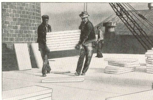
Easy to handle. Two men here carry 8 Kaylo Roof Tiles, walking on roof deck already laid.
