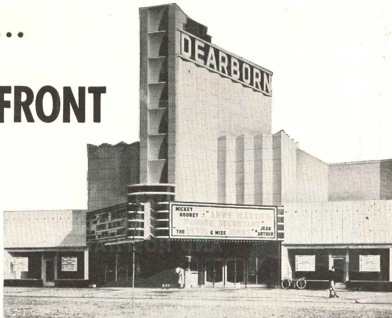
Inconel clips hold this facade secure! Specified by the architects, Charles N. Agree, Inc., colored Glasiron panels provide a permanently attractive appearance for the Dearborn Theatre, Dearborn, Mich. For more information about Glasiron, write: Wolverine Porcelain Enameling Co., Detroit, Mich.
