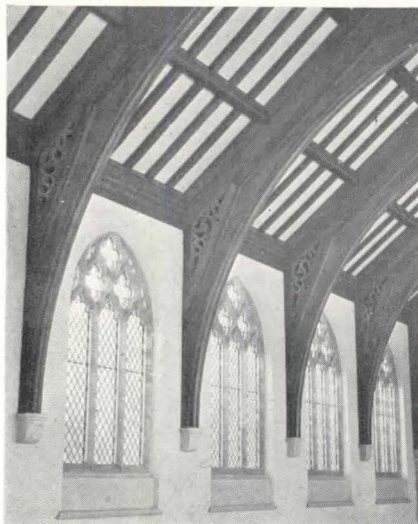
Acoustical board of wood fiber applied between rafters and purlins; Grace Lutheran Church, Fremont, Ohio; Cram and Ferguson, Architects. (Right) Vaults and wall spandrels faced with acoustical tile in Church of the Holy Child, Phila.; George I. Lovatt, Architect
