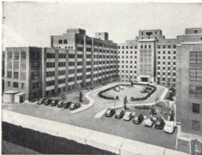
Delaware Hospital, Wilmington, Delaware. Heated by 6-zone Webster Moderator System of Steam Heating. Completed in 1942. Unit No. 1, center, occupied in 1940. Architects: Massena & duPont, Wilmington. Consulting Engineers Jaros, Baum & Bolles, New York. General Contractor: Turner Construction Co., Philadelphia. Heating Contractor: Benjamin F. Shaw Co., Wilmington.
