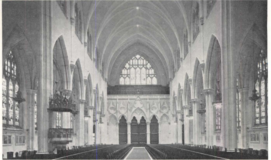
To reduce reverberation, wall ashlar is surfaced with structural acoustical tile, and vaulted ceiling with acoustical plaster in St. Joseph's New Cathedral, Buffalo; Eggers and Higgins, Architects. Here, acoustical plaster is a weight-saving factor
