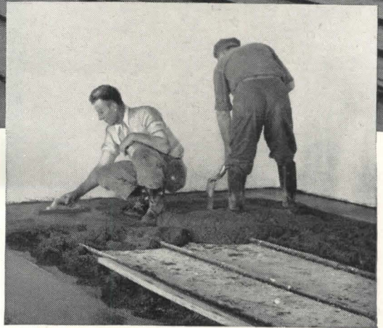
Covering coils with a topping of ordinary concrete
