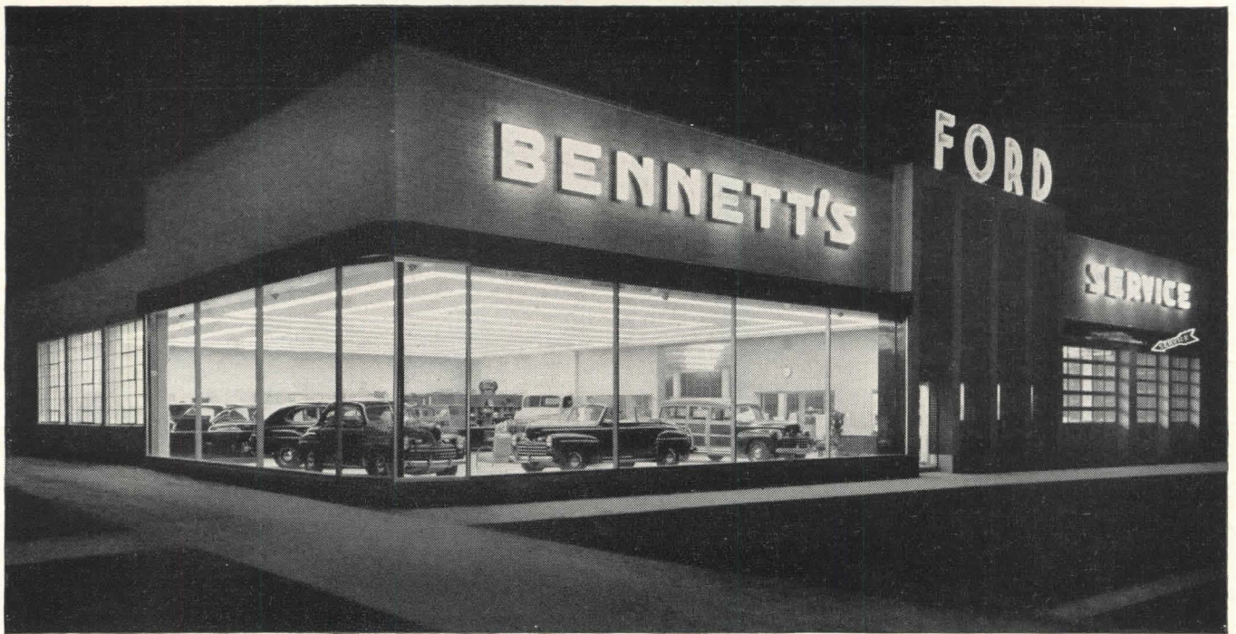
VISIBILITY OF THE ENTIRE SHOWROOM is made easy by large plate glass windows on front and side. The showroom is flooded with daylight—and at night exhibits the autos in a brilliantly-lighted, giant showcase.
