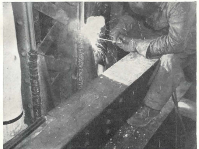
Fig. 3. Brackets from 21-inch I-beam are welded to existing column.
