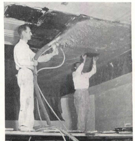
(Left) Perforated acoustical tile being applied with adhesive to plaster face of vaulted ceiling. (Center) Another treatment of warped surfaces is with rockwool tile resembling travertine. (Right) Sound-absorbing asbestos fiber can be sprayed on prepared surfaces
