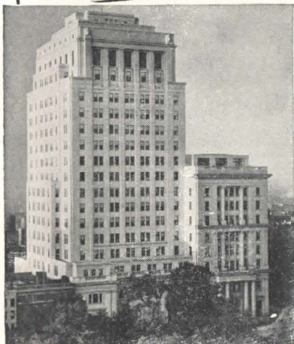
THE PENN MUTUAL LIFE INSURANCE CO. Home Office, Philadelphia, Pa. 10-story building at right built 1914. 20-story addition built 1933.
