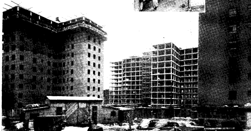
Truscon Diamond Metal Lath Used in Elliot Housing Project, New York City.
