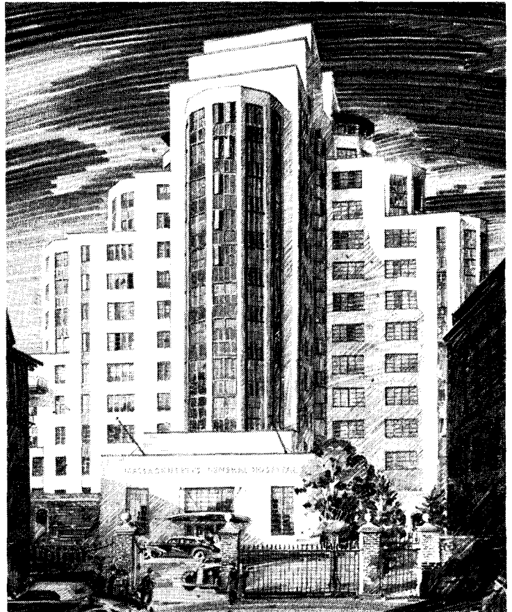
GEORGE R. WHITE MEMORIAL BUILDING MASSACHUSETTS GENERAL HOSPITAL Architect: Coolidge, Shepley, Bulfinch and Abbott—Boston, Mass. Engineer: Office of Hollis French—Boston, Mass. Contractor: James S. Cassidy, Inc.—Cambridge, Mass.
