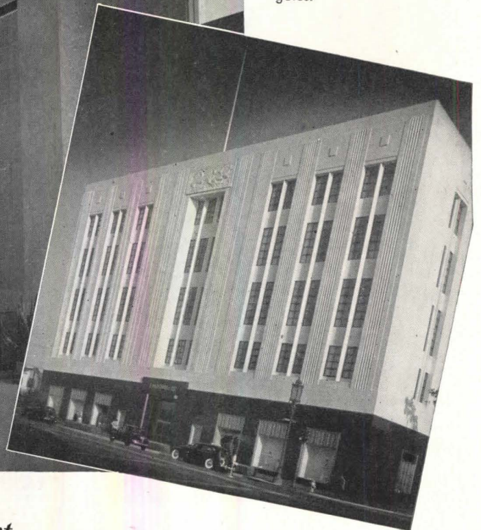
(Below) Marble and polished black granite façade of the store, built by William Simpson Construction Co., Los Angeles.
