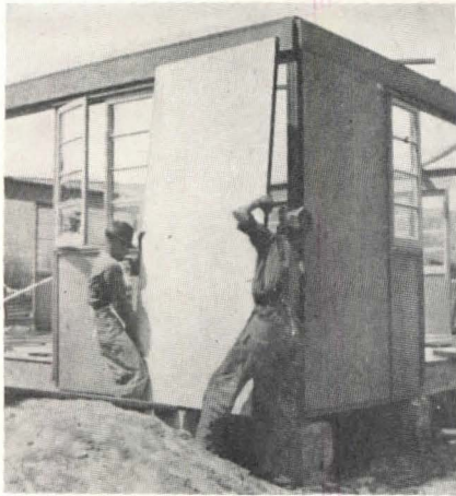
Insertion of insulated wall panels in a prefab. From "The Prefabricated House"
