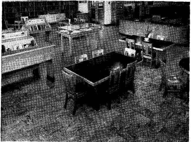
In libraries and other classrooms where noise should be held to a minimum, rubber tile is frequently preferred because of its high resilience. Cork tile, often rated the highest in resilience, requires more than average maintenance. Where cost is important, linoleum is suggested.
