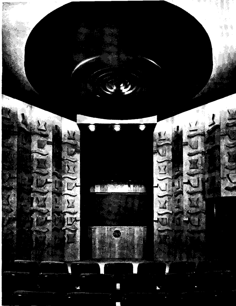
LEFT: Front of theater has a stage that more often presents equipment rather than people. Sound-absorbent dropped panel above stage carries spotlights; general indirect light by incandescent bulbs on hung soffit is controlled by electronic dimmer. RCA emblem conceals 10-in. loudspeaker which connects with sound-film projector at rear for theatric programs
