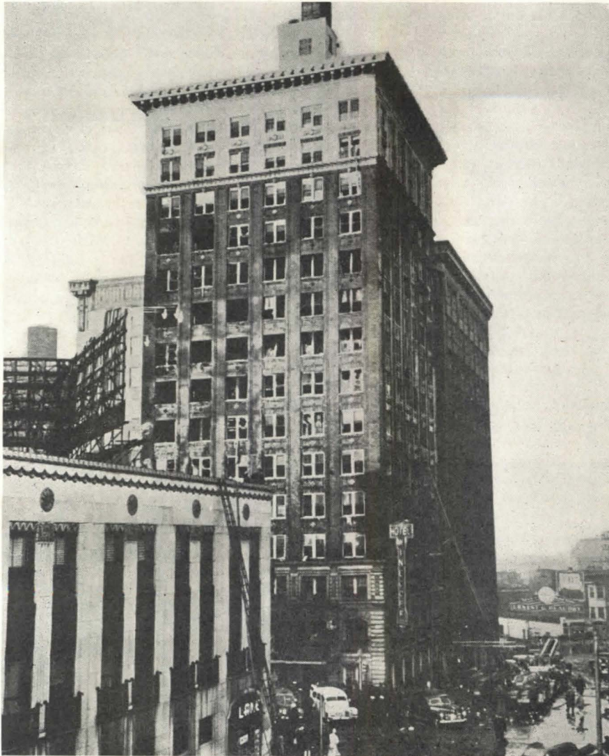
119 persons died in the Winecoff Hotel, Atlanta. Erected in 1913 of fireproof construction, it had only a single exit stairway, open and unprotected from the flames that roared upwards from the point of fire's origin in the third floor corridor. Combustible trim and furnishings fed the flames, and open transoms turned guest rooms into fire traps
