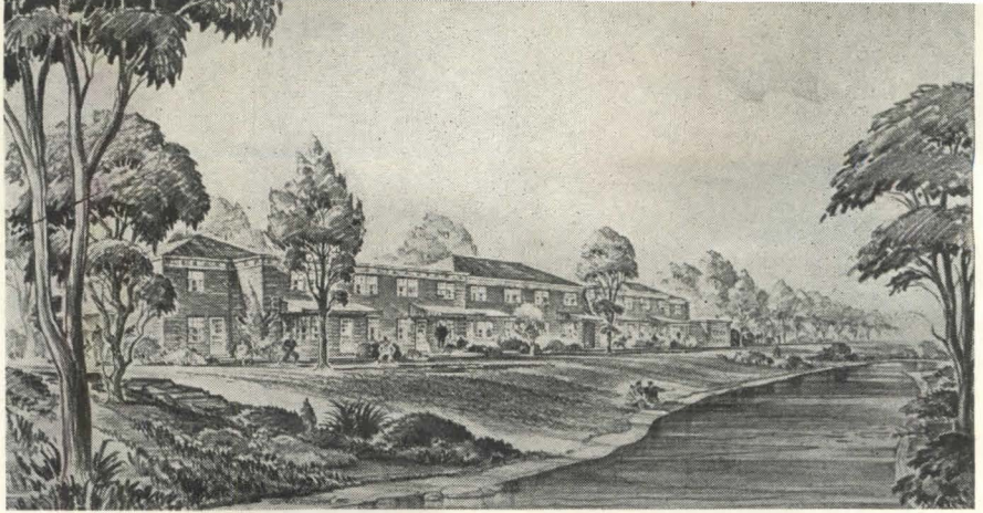
Waverly Apartments, for Savings Banks Trust Co., Harrison, Ballard & Allen, Architects
