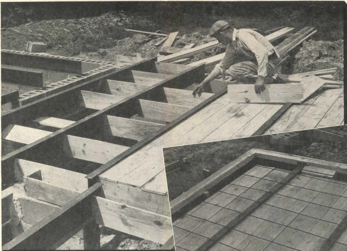
Spreaders are placed about 30" to 36" centers. A few nails hold the four 8" form boards in place. The boards can be used later as roof sheathing. Concrete will encase ends of beams to provide a fire stop and support for a bearing partition.
