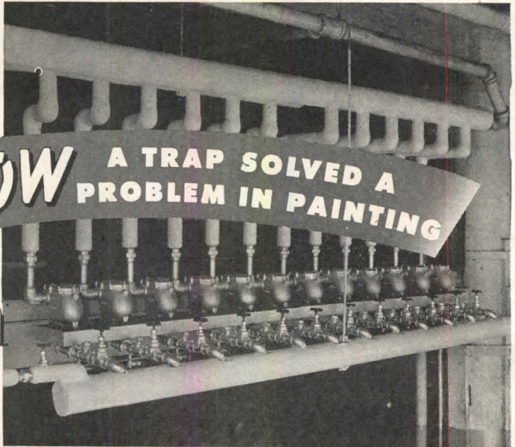
Above: Twelve Class 200 Industrial Float Traps, connected to high pressure steam heating coils in paint drying ovens in the Ford Rouge Plant. Left: Cutaway view of the Trane Class 200 Industrial Steam Trap, which Trane furnishes the Ford Motor Company.
