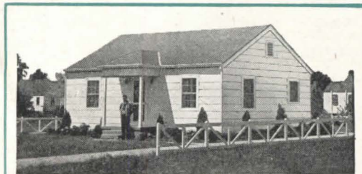
Aluminum requires no protective surface coating. However, it may be painted for decorative purposes, as in this house constructed with Reynolds Lifetime Aluminum Building Products.
