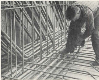
Steel bars for reinforcing concrete feature reverse helical ribs for an improved bond
