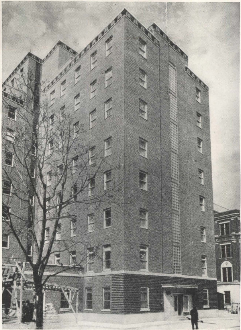
Eight stories in height, this 50 bed, solarium-equipped addition to the New Rochelle Hospital, New Rochelle, N. Y., used 32½ tons of Bethlehem Open-Web Joists. Contractor: Turner Construction Co., New York. Architects: Shreve, Lamb & Harmon Associates, New York.
