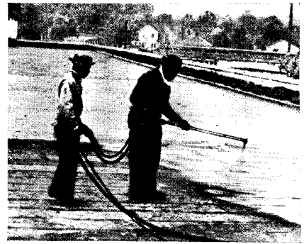
Faster roof-coating by cold-spray method
