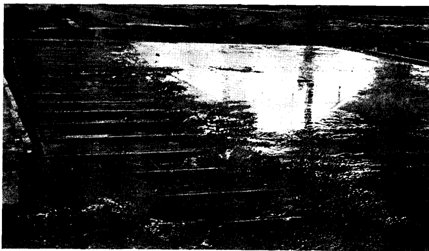
Radiant-heating coils form an integral part of the floor. Cement is poured on a 12-in. fill of compacted gravel. Before pouring, pipe joints are pressure-tested for leaks
