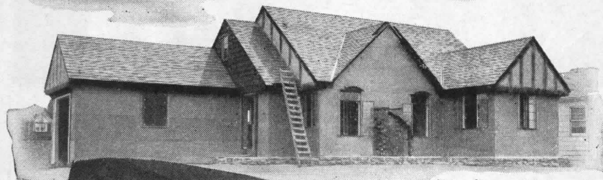
Note absence of batten strips and tears in this SISALKRAFT application. This reinforced paper is strong enough to pull around corners.
