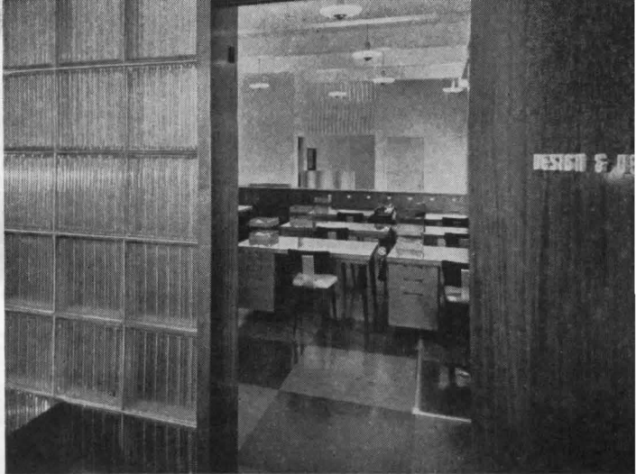
View through general office looking toward reception room
