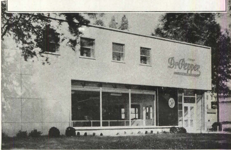
Dr. Pepper Bottling Plant, Kinston, N. C. Thin, precast Architectural Concrete Slabs made with Atlas White cement by Arnold Stone Co., Greensboro, N. C. Facing is white; name in red vitreous aggregate is cast in the slab. Architect: John J. Rowland, Kinston, N. C. Contractor: H. L. Coble, Greensboro, N. C.
