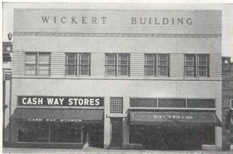
ARCHITECTURAL CONCRETE SLABS applied over old brick finish on the Wickert Building, Escanaba, Mich. The facing is buff; base course is green; and the monolithically cast raised letters are in green vitreous aggregate. The matrix is Atlas White cement. Architects: Hubert & Gjelsteen, Menominee, Mich.; Contractor: Mike Rettman, Bark River, Mich.; Slabs by Badger Concrete Co., Oshkosh, Wis.
