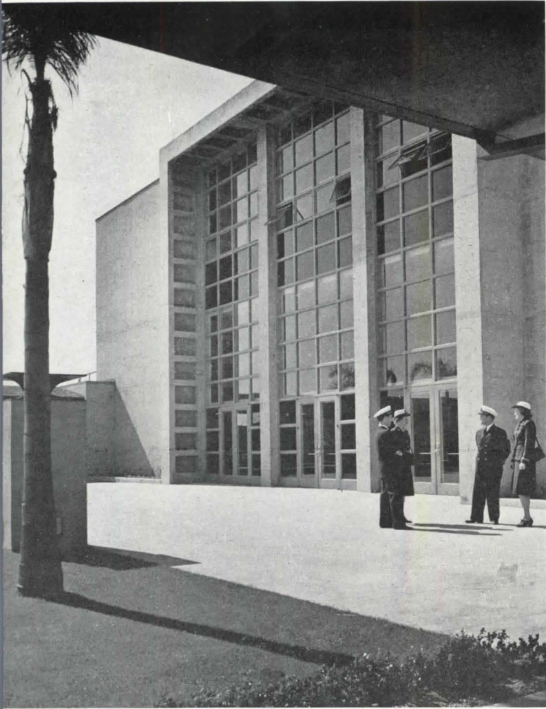
Opposite page and left: views of main entrance of auditorium-gymnasium from various positions in the open court. Note massive concrete pylons capped with metal reflectors, forming indirect light standards. They give a subdued lighting in the patio
