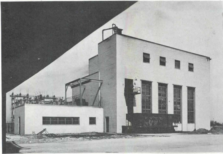
Boiler house for the Thompson Aircraft plant at Cleveland. This is a typical wartime boiler house providing steam and compressed air. But electrical power is purchased; note transformer substation, left rear
