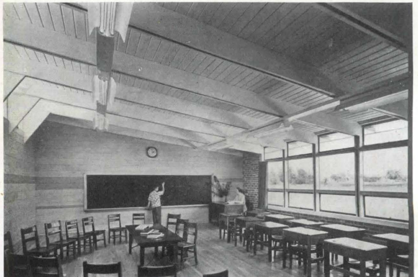
F. Similar to E, above, but in a more northerly location and with reversed orientation. Fc readings, taken at noon, August, in room facing E, ranged from 100 or more to 60; in activity alcove, 100 or more to 20. Facia board held out from building on outlooker helps to shade the main windows in the morning, reflect afternoon sunlight into them
