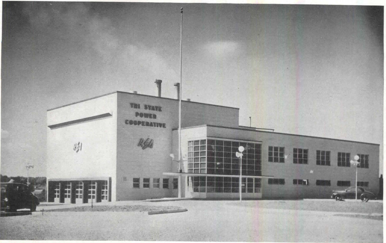
The Dairyland (formerly Tri-State) Power Cooperative, one of the prewar REA plants. Roland A. Wank, architect; A. Y. Taylor & Co., engineers
