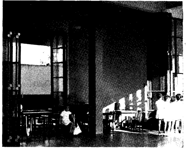
High glazed doors fold back for light, air and ventilation
