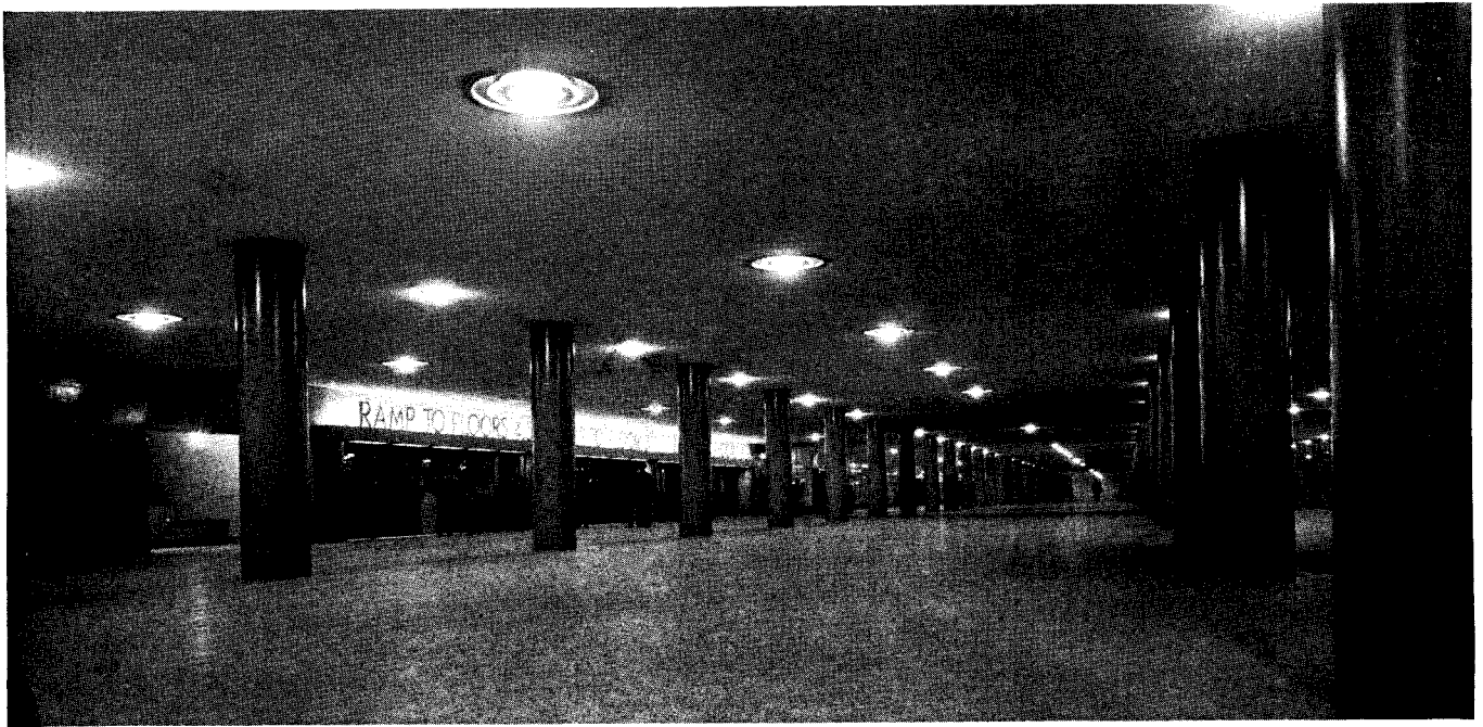
Above: The concourse, a forest of red columns between walls of glazed terra cotta, is 680' long. The ceiling height is 10'-11 1/2"
