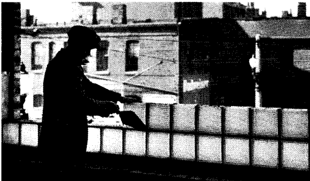
Any competent bricklayer, using regular equipment, can lay up INSULUX Glass Block panels. Little or no metal is needed for replacement panels like this one.
