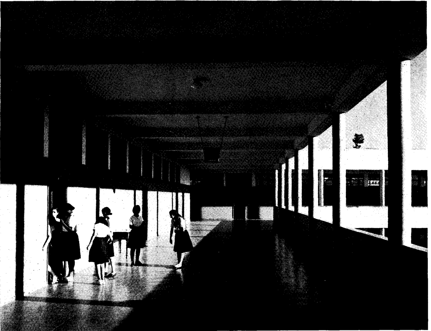
Wide covered porches serve both for circulation and for outdoor activities in inclement weather
