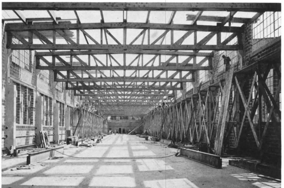
With the structural elements precast, walls and roof require minimum labor
