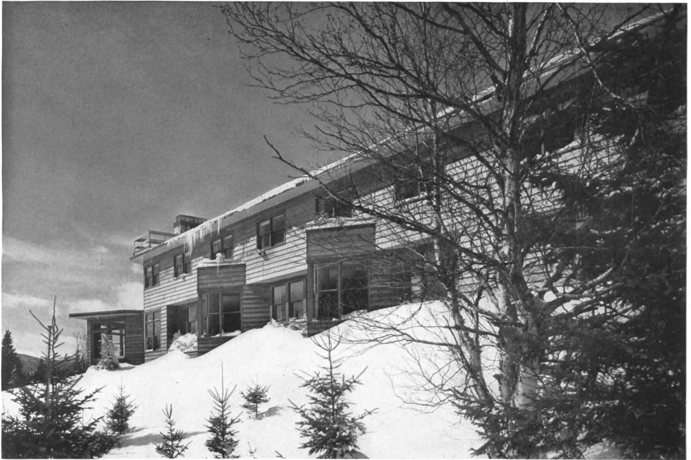
Form follows function in the design of the v-shaped alcoves which add interest to the facade and admit full sunlight to the classrooms
