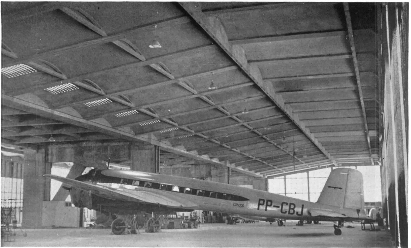
Above. Interior of hangar looking toward the glazed end. The widely spaced columns support longitudinal trusses which carry the cantilevers. Ceiling is formed by segmental roof arches on lower chords
