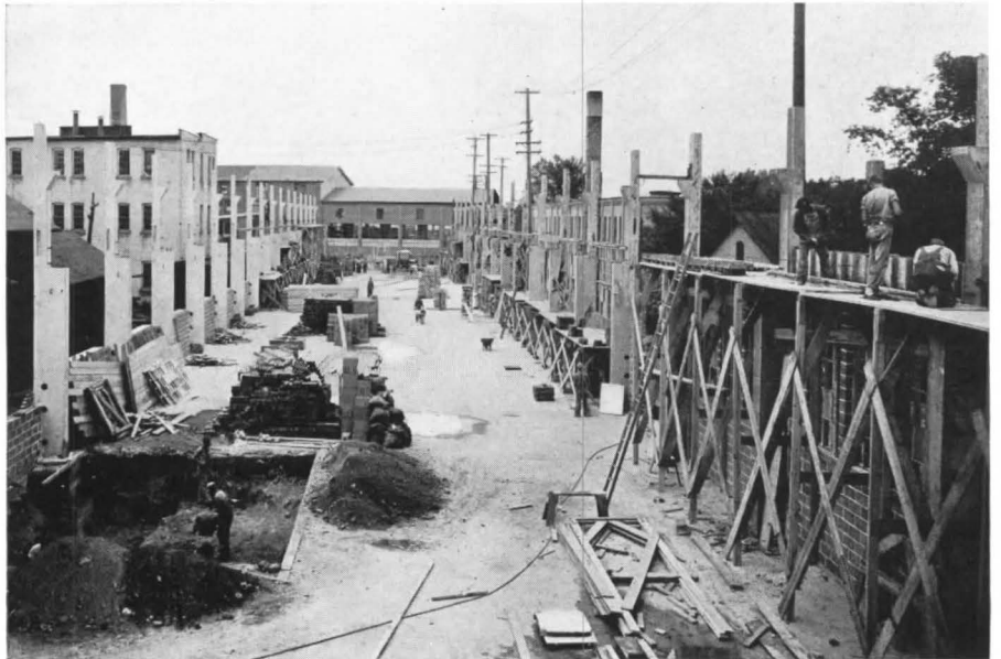
With the columns set in place, work can proceed quickly at all points
