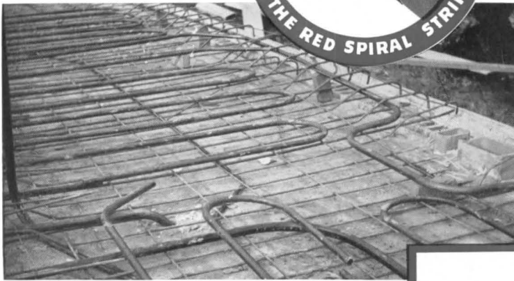
NORTH HILLS LIBRARY, Pittsburgh, Pa. FRANKLIN & BROWN, Architects E. S. TOWER, Engineer
