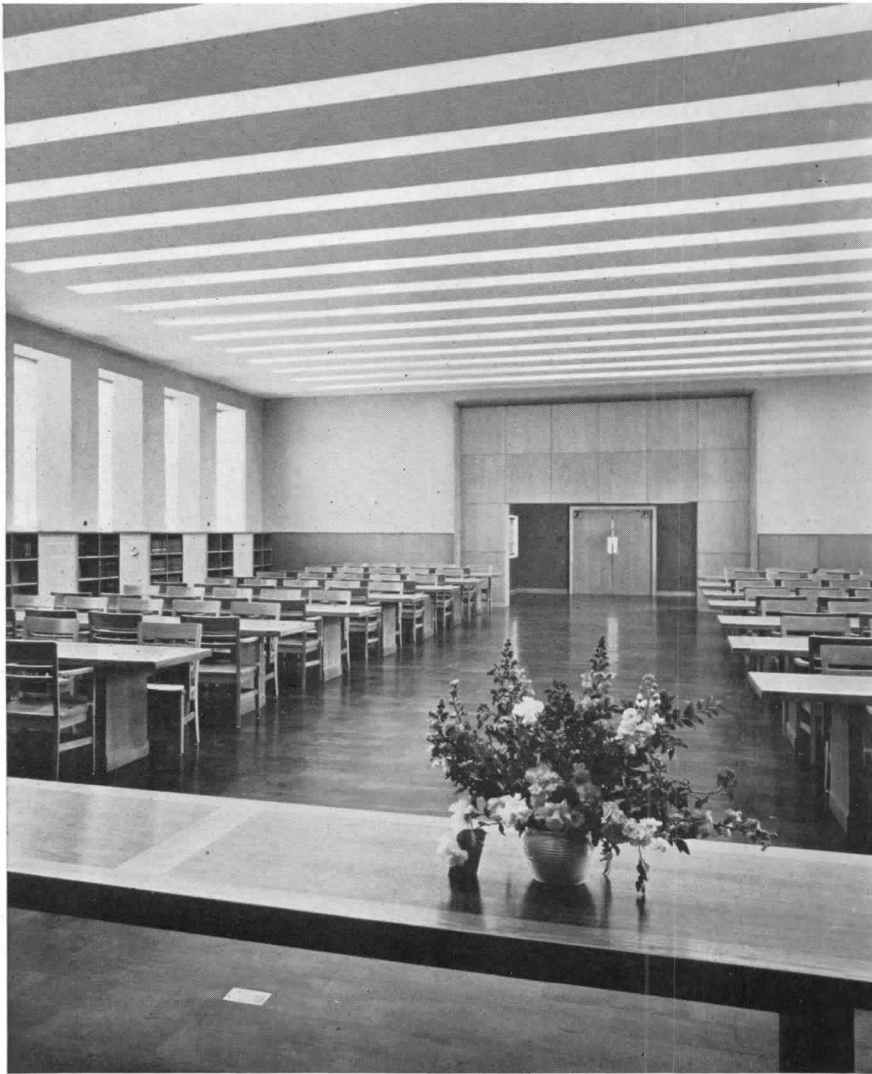
LIBRARY. Acoustical ceilings; fluorescent light, flush mounted
