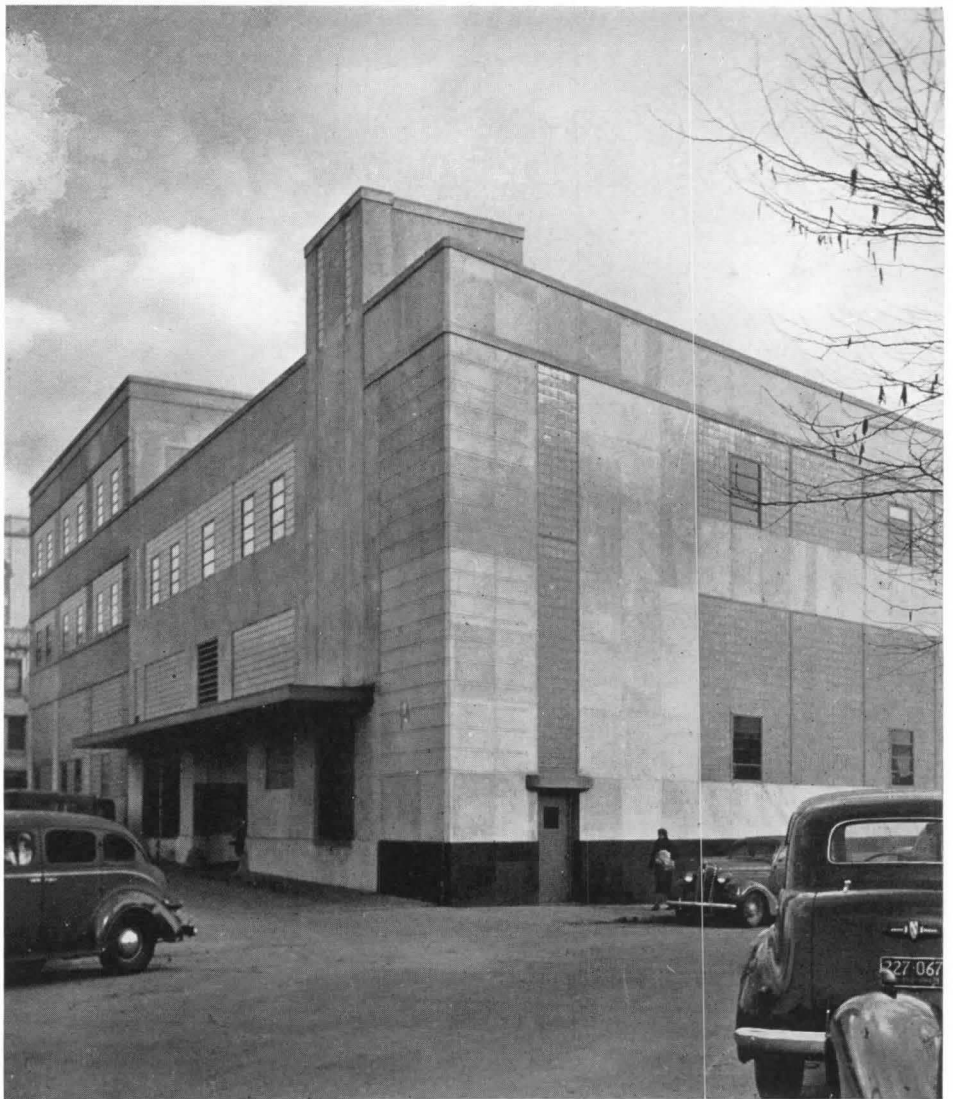
REAR VIEW. Advantage was taken of the site slope to the rear for simplifying the handling of stores of newsprint and ink, a very considerable item. From the truck-bed-high loading platform near the rear of the building, paper goes to the basement on an electrically operated paper drop. Thereafter it is handled horizontally on dollies running on trackage sunk below basement level (see basement floor plan) either to storage room or reel room from which the press is serviced. Space is provided for a month's supply
