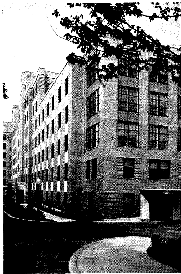
Photos, left to right: exterior; main entrance; clinic entrance; lobby, Unit 1; clinic lobby, Unit 2. Structure has reinforced concrete skeleton, brick walls shaded progressively lighter from base to coping, limestone trim. Color is extensively used in operating rooms, public and private bed spaces. All possible means of noise control are employed; sources are eliminated or acoustically treated; installation of sound-deadening material is called largest in any privately financed hospital. Signal system operates lights instead of loud speakers or bells
