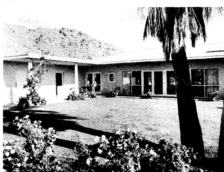
EXTERIOR PLASTER WALLS are coral in tone; the roof is of tan tile
