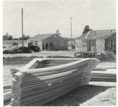
Standardized mass production on the site, for FSA farm homes, unimpeded by building codes
