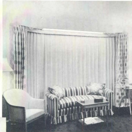
Illuminated soffit gives general illumination of room at night same general direction and distribution as in daytime
