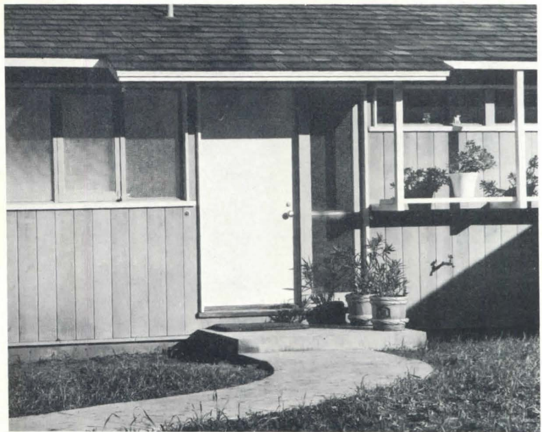
This entrance meets most requirements for safety — indirect lighting, solid wood door, protected platform and step, minimum number of steps. Door sill might have been somewhat lower, since average person does not expect a change in floor level which comes right at door. John Ekin Dinwiddie, Architect
