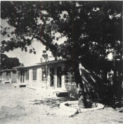
Contrast Fort Greene Houses, Brooklyn, N. Y. (W. F. R. Ballard, Consulting Archt.), with Rosewood, Austin, Tex. (Page & Southerland). Three groups of associated architects are collaborating on different sections of Fort Greene
