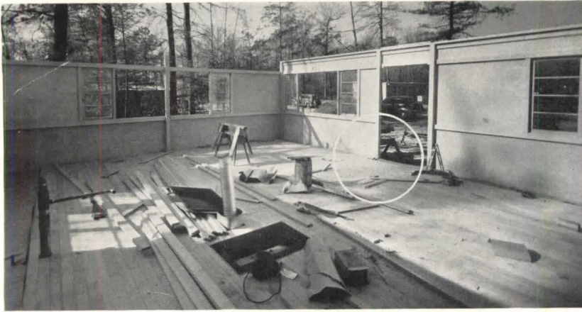
Interior view of wall elements in place
