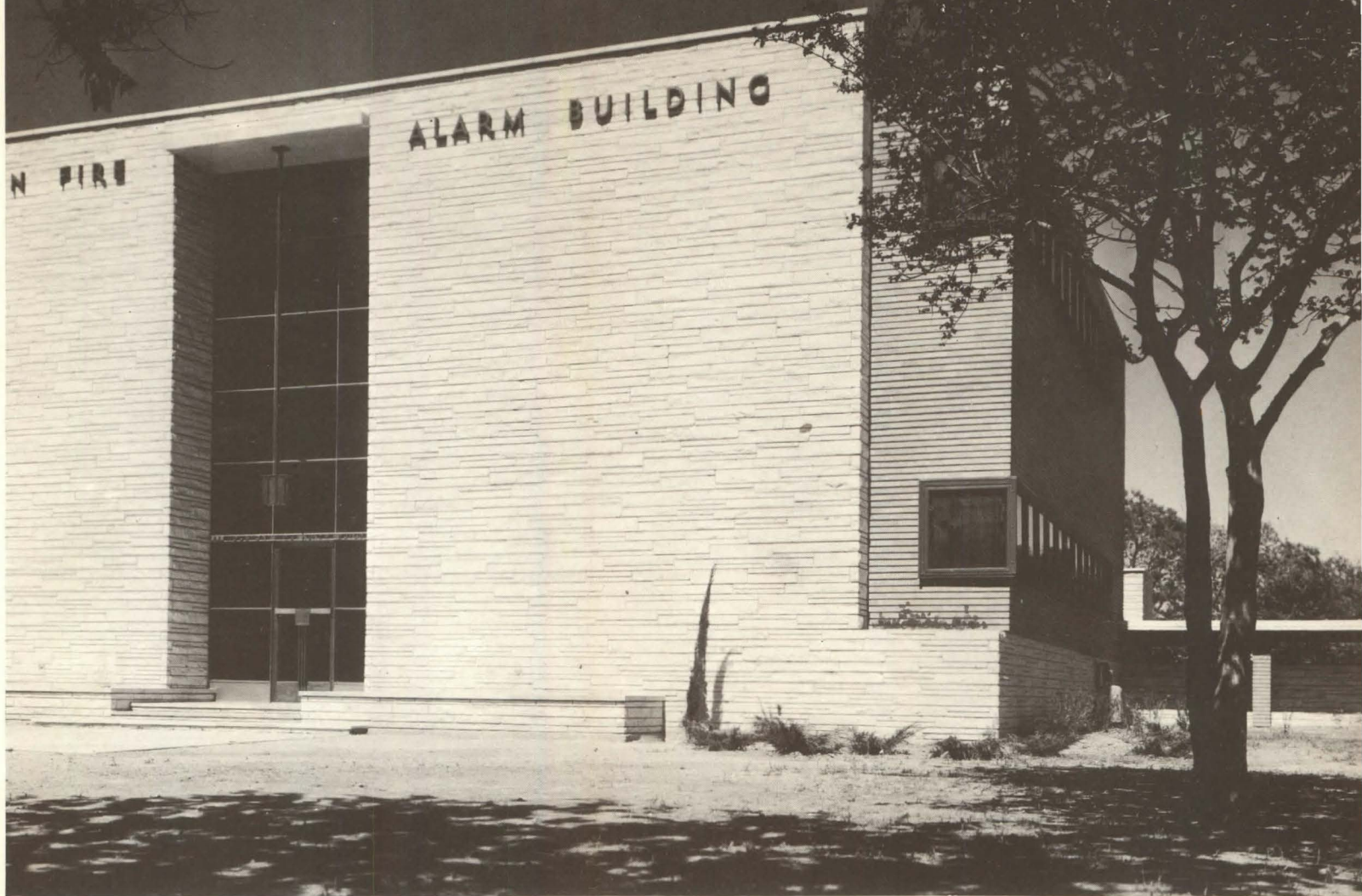
Mackie & Kamrath, Architects: Central Fire Alarm Building (above) and repair shop (right) for Houston, Texas.
