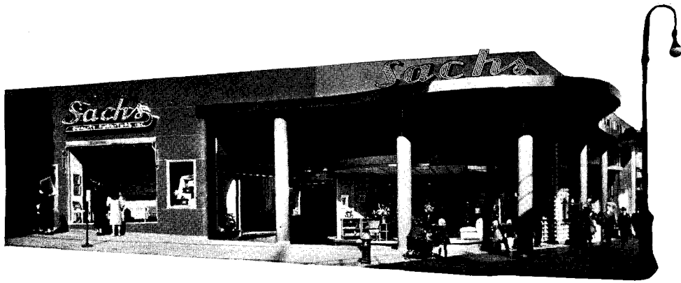
SACH'S small department store, New York City; MORRIS LAPIDUS, Architect, FRANK S. PARKER, Associate Architect. Many kinds of merchandise, each in a specially designed window, had to be displayed in a single front
