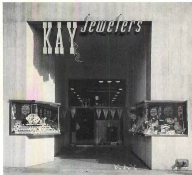
ARCADE for narrow frontage; Kay's, Knoxville, Tenn.; MORRIS LAPIDUS, Architect for ROSS FRANKEL, INC.
