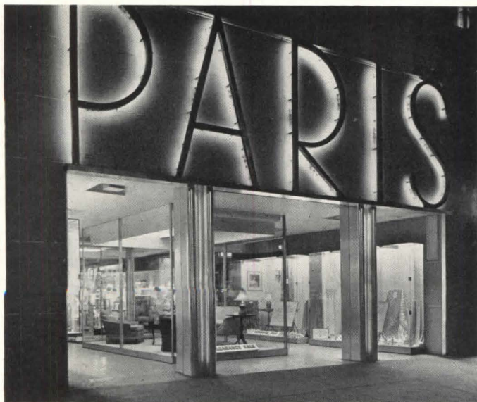
LARGE LOBBY, Paris Decorators, New York City; MORRIS KETCHUM, JR., Architect; GRUENBAUM AND KRUMMECK, Associates
