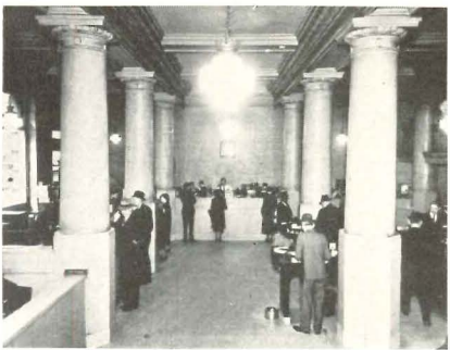
OLD (below) and NEW main banking room
