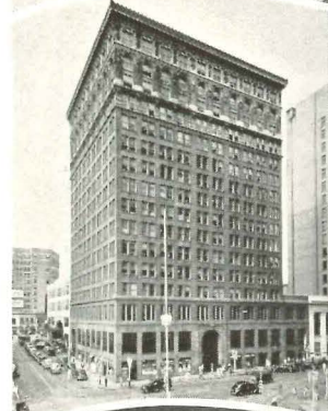
First National Bank Bldg., Atlanta, Ga. Newcomb & Boyd, consulting engineers, Atlanta. Atlanta Office of York Ice Machinery Corp., air conditioning.
