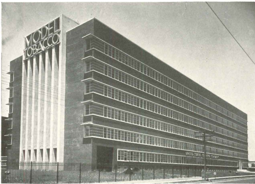
ELEVEN NOMINATIONS: United States Tobacco Co. Model Factory. It was designed by the architectural firm of Smith, Garden & Erickson.
