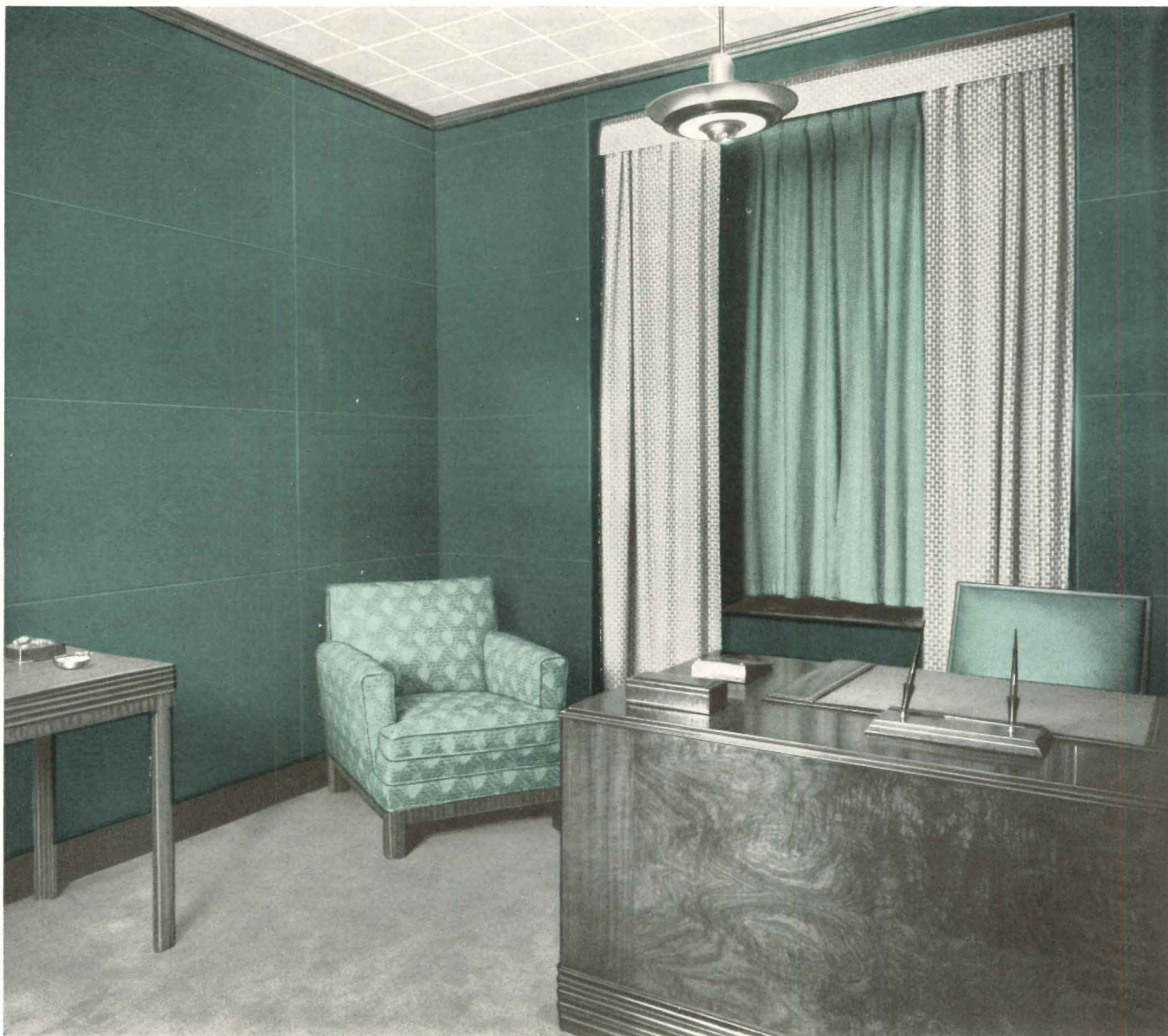
Vinylite veneer on Transite Walls forms an attractive finish in this executive office.
