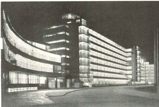
Fig. 3: AT NIGHT THE RIBBON WINDOWS do not light the factory, but the street. Looks fine, but a tremendous amount of light is wasted.
