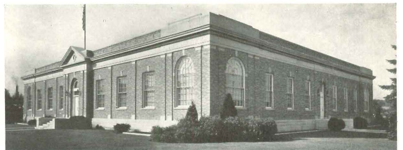
FOUR NOMINATIONS: new research laboratory of the American Tobacco Co. It was designed by the architectural firm of Francisco & Jacobus.
