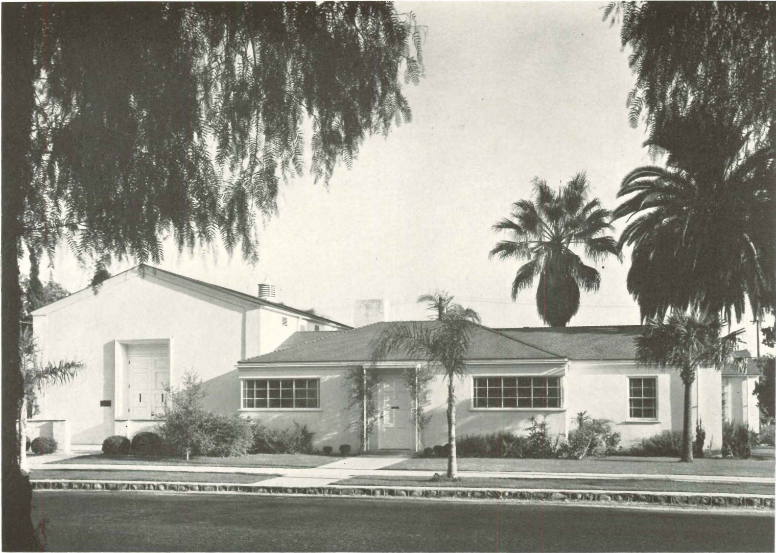
THE TWO ENTRANCES clearly define the chapel and the business office. Families may reach their room privately through the patio.
