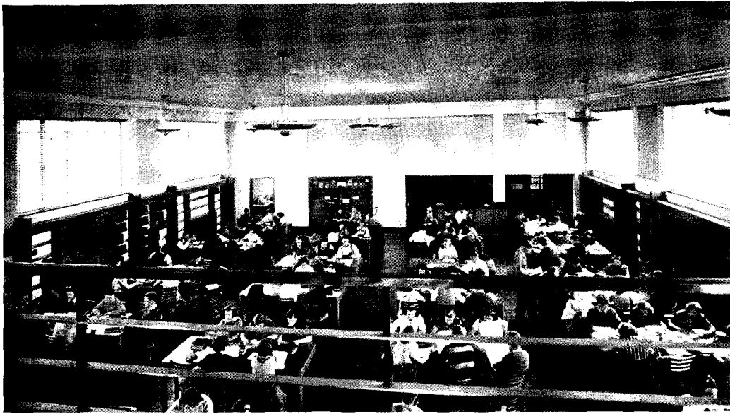
Library, looking from balcony, below which are conference rooms. Charging desk (upper right) is at main entrance.
