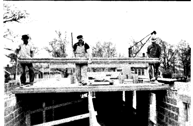
Fig. 7. Increasing variety of shapes in hollow tile yield possibility of prefabricated reinforced members. Typical unit employed (top) in prefabricated beams (bottom).
