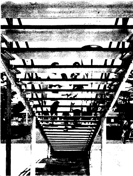
The Glass Center features treads of toughened glass on metal stringers.
