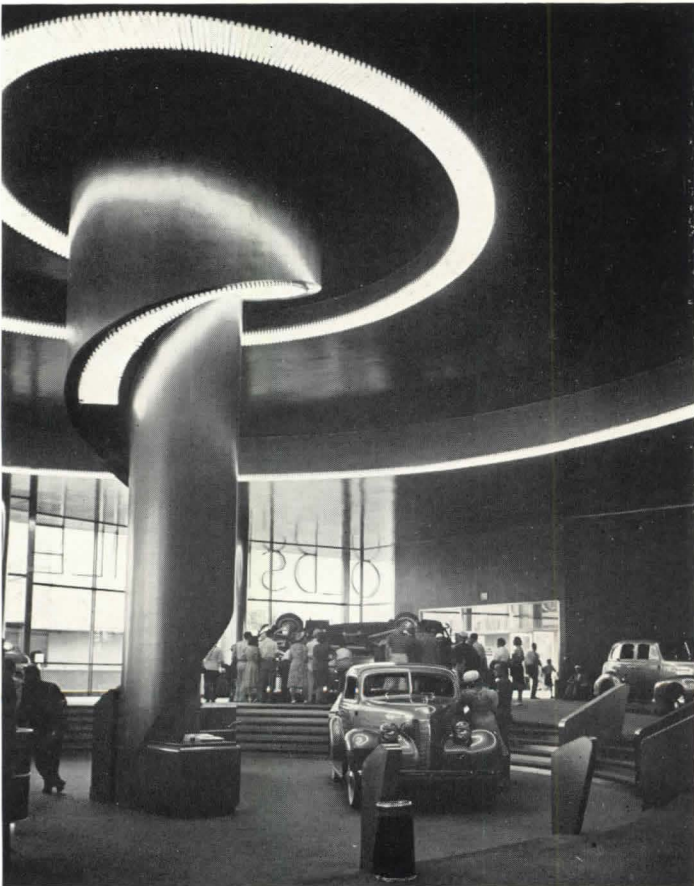
Fluorescent tubular lamps, mounted side by side, are spiraled around the central post in a General Motors' salesroom.
