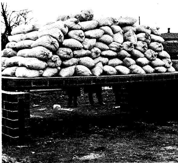
Fig. 2. Reinforced tile beam and slab, designed for a load of 50 lbs. per sq. ft., with 180 lbs. per sq. ft. Similar tests ran up to 720 lbs. per sq. ft.
