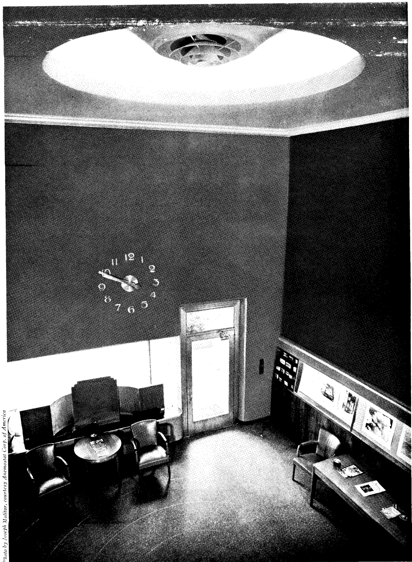
Office of American Airlines. Harrison & Fouilhoux, Architects. Anemostat is combined with trough lighting.
