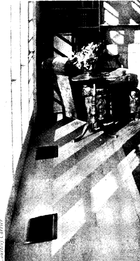
5. Floor outlets near an exposed wall counteract the cold air which sweeps down the outer wall and across the floor.
