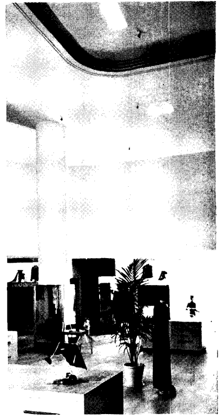
3. Space between ceilings and floors above is a plenum chamber; most of the lamp heat is carried off in air outflow.
