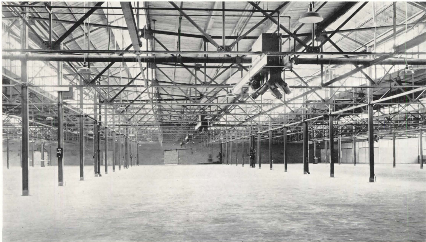
A wide one-way span employing a more conventional type of structural framing. Even distribution of daylight from monitor sash results when the monitor is 2.4 times the width of the valley bay measured at the top of the monitor. The interior of the Star Box and Printing Company plant at Chattanooga, Tenn. The H. K. Ferguson Company, engineers and builders.
