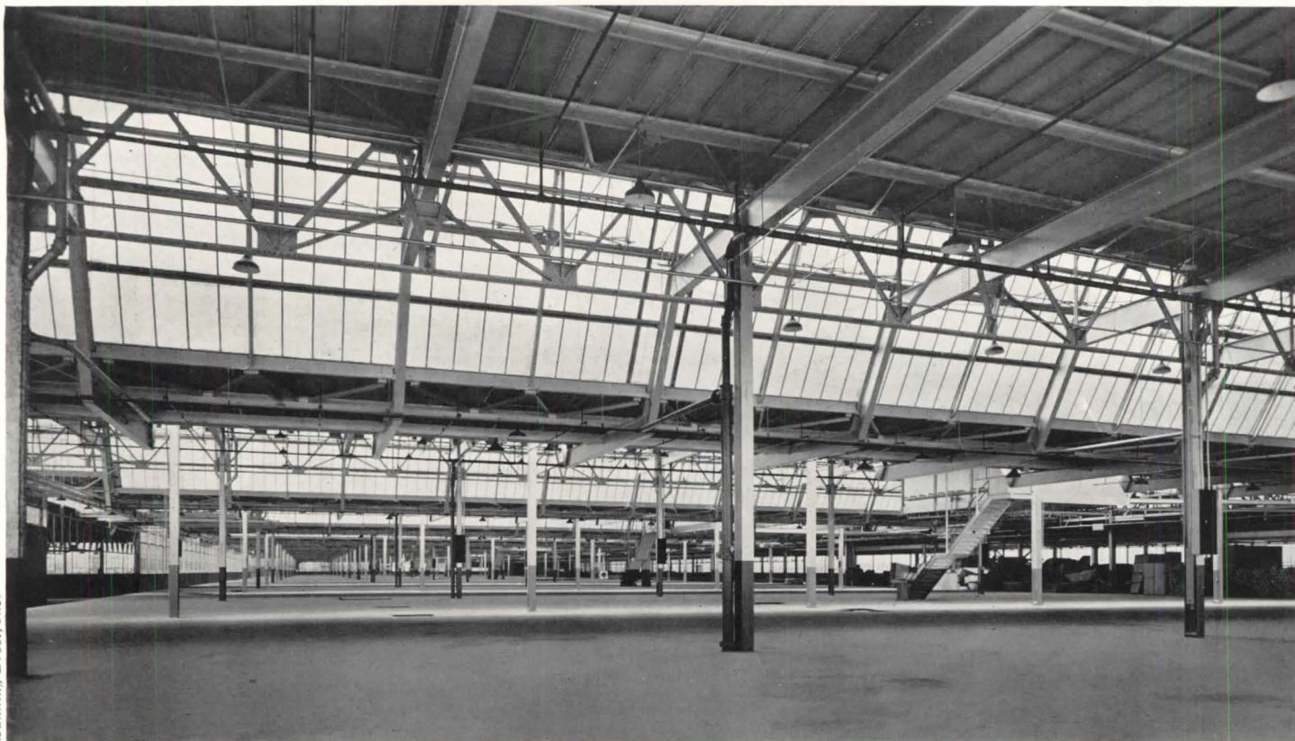
Wide column spacing—40 by 60 ft.—leaves floor space unobstructed and promotes flexibility in plant operation. By designing roof beams as cantilevers over supporting columns the weight of structural steel per sq. ft. is no more than would be required if column spacing were 40 by 30 ft. Picture shows part of the interior of the Dodge Truck factory in Detroit for which Albert Kahn, Inc., was architect and engineer.
