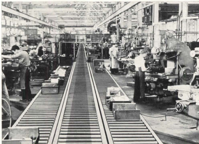
A live-roller conveyor in the center carries parts of electric motors between distant machine operations of a large plant. Flanking conveyors simplify straight - line handling of parts requiring a succession of related operations.
