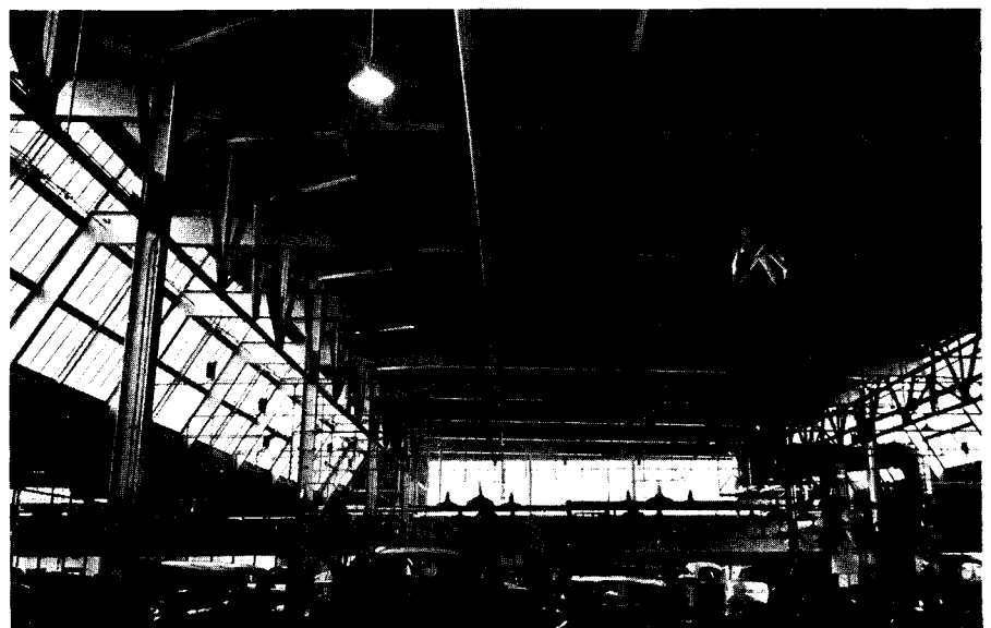
Main assembly line, showing some of the fifteen hundred 450-w. mercury lamps.
