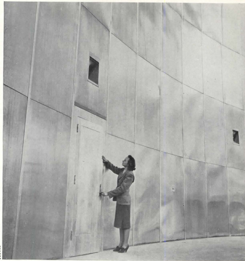
Acme Air Conditioning Mt. Palomar observatory. Between inner and outer aluminum-plate walls is a 4-ft. plenum chamber.
