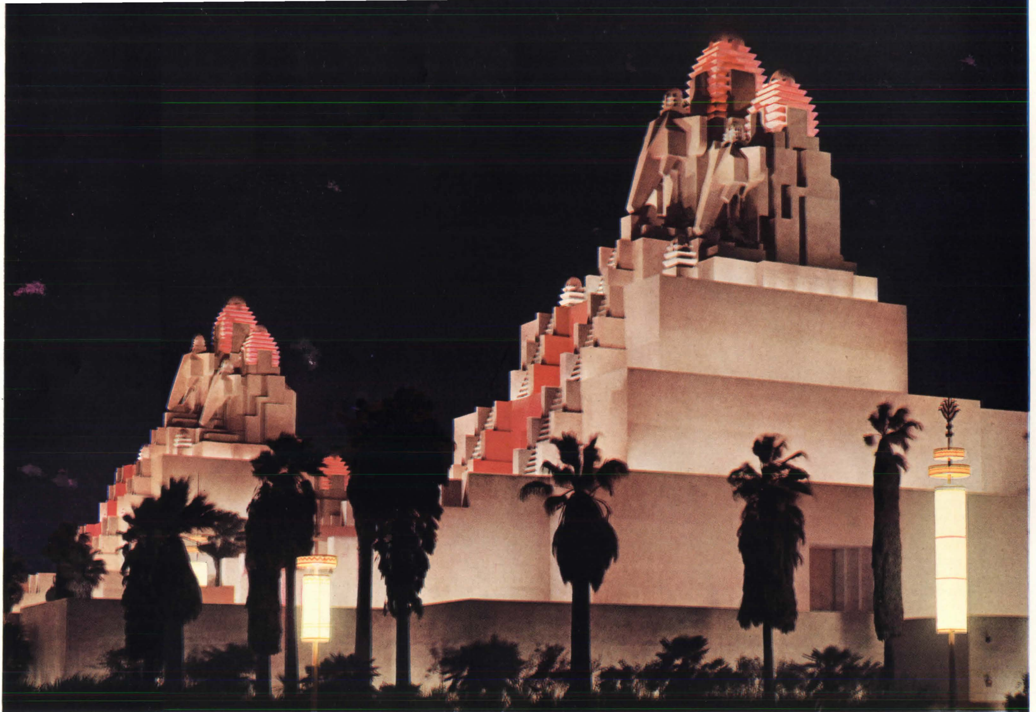
PLATE 5. Highest intensities and lightest colors have been widely used on those elements primarily designed to be seen from afar. Thus the brilliantly lit West Facade, with its monumental entrances, actually serves as a huge sign which dominates the city's eastern horizon and intersects its traffic lanes to the mainland. Colors are concentrated at the entrances.
