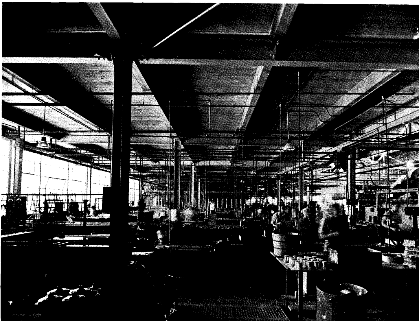
Plating Department: Acid-bath fumes caused wood roof deck to be used; on steel framing only is periodic painting needed.
