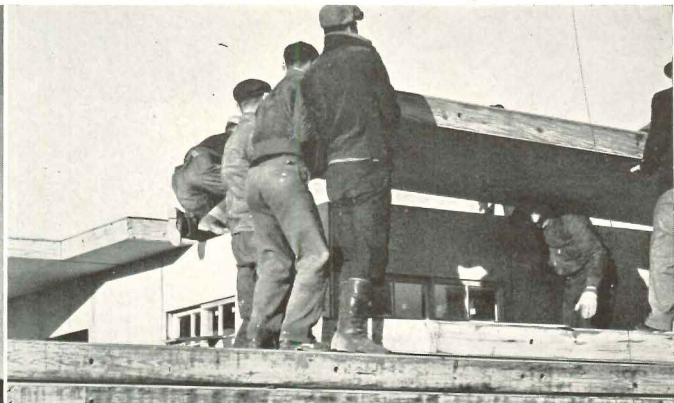
8. When the walls have been completely assembled and bolted together, the roof panels are placed in position.
