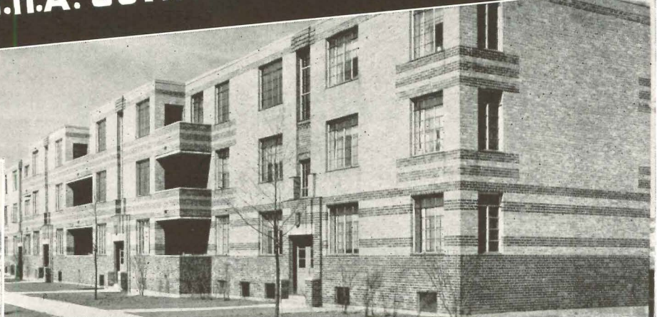
Outhwaite Homes, U. S. H. A. Housing Project, Cleveland, Ohio.
