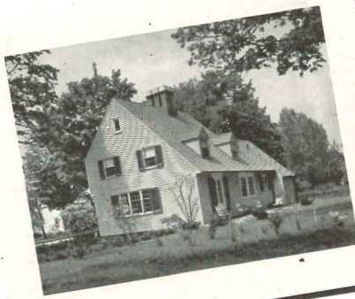
Architect, Willis Mills, New York City
