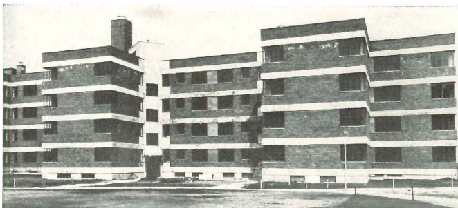
• The Ten Eyck (Williamsburgh) Housing Project. A 50,000-yard installation, of Milcor Solid Plaster Partitions in Buildings 1, 2, 3, 4, 6, 7, 8. Photo courtesy of FHA.
