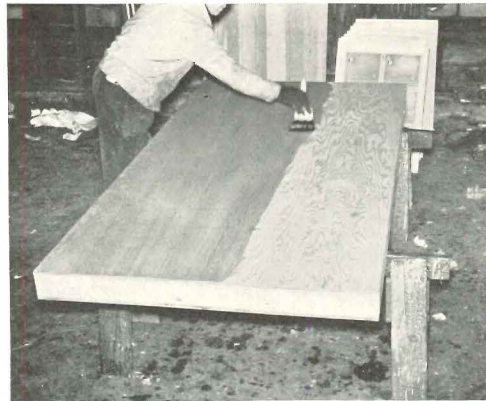
3. Panels are sized with Tung oil. Painting is done after house is assembled. . . .
