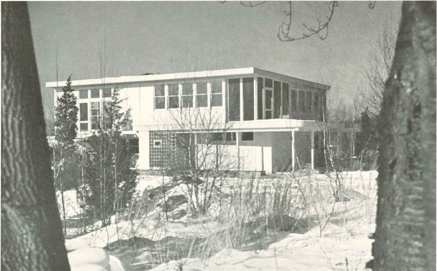
View from south. The room above the covered walk is a nursery, with ready access from sleeping porch and master bedroom.
