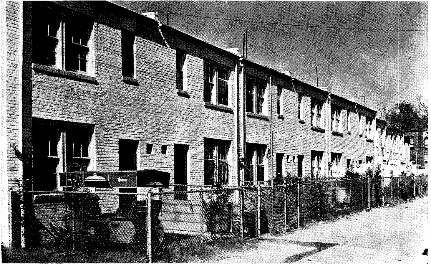
Rear view of new dwellings. One of two wings extending from the street back to a row of remodeled alley dwellings.
