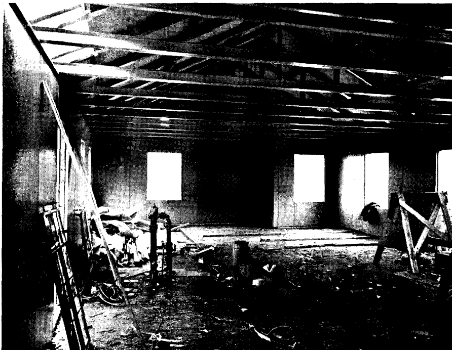
Exterior walls and ceiling are 1-in. metal-sheathed panels; a standard metal joint system and crack filler give interior finish without molds or battens (left).
