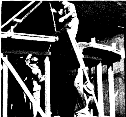
4 Forms in place, reinforcing begins . . .
