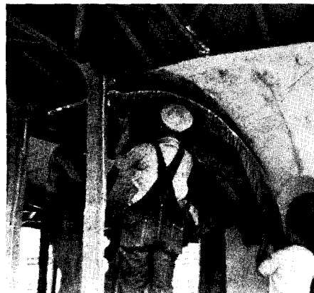
10 Then formwork is removed . . .
