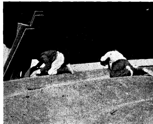
11 top surface waterproofed . . .
