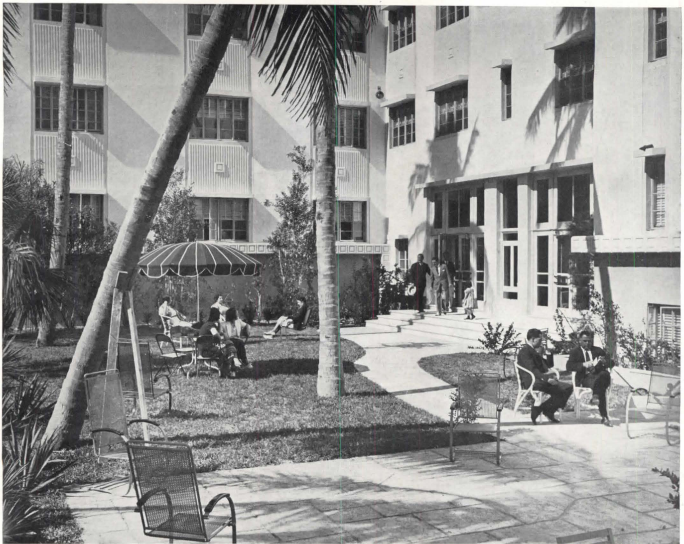
View of Patio and Lounge Entrance
