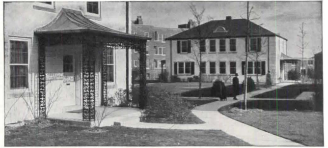
Smyser-Royer cast iron verandas used on operation-built dwellings add a note of charm to simple design. Buckingham Community, Arlington, Va.
