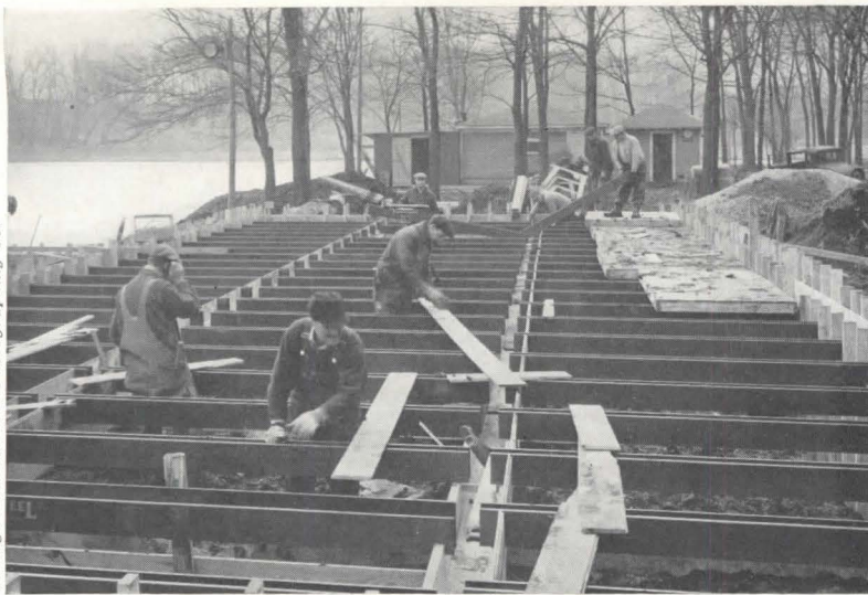
THE STEEL SECTIONS SHOWN ABOVE ACT AS FORMS for poured-in-place concrete beams on which rest lightweight concrete precast slabs. The slabs are laid in a
