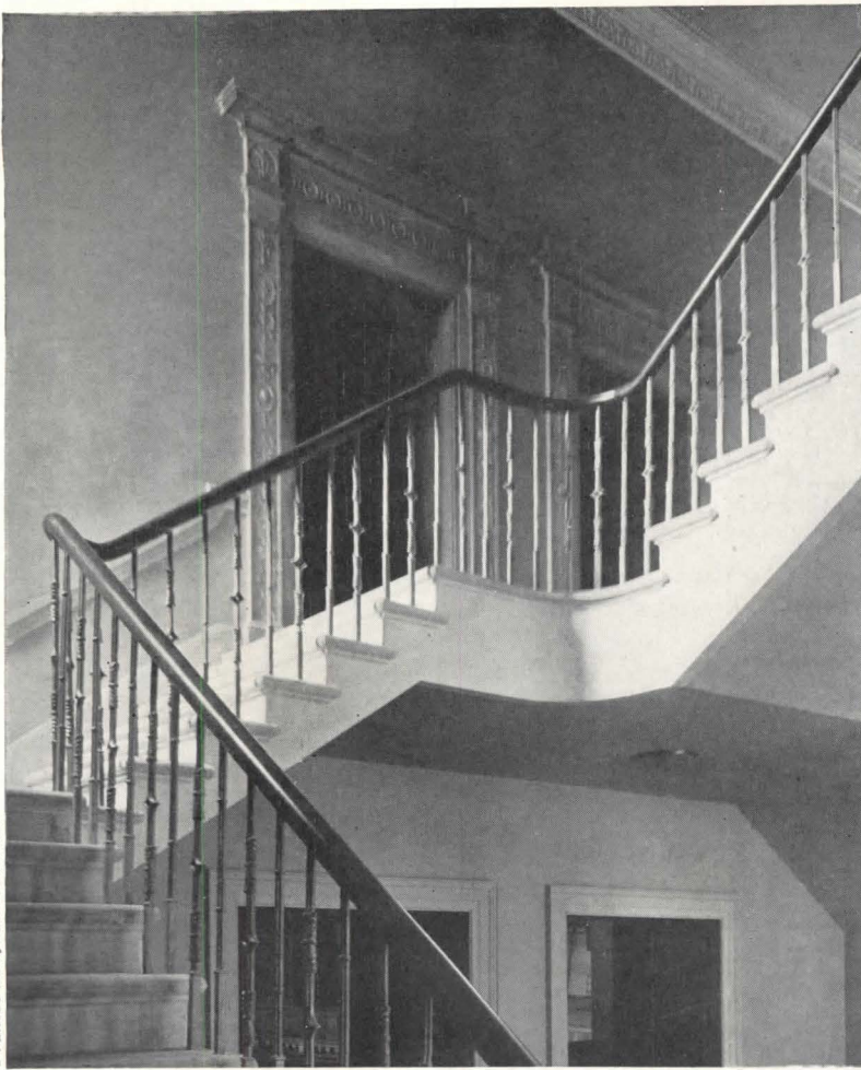
Main Stairway, rebuilt
