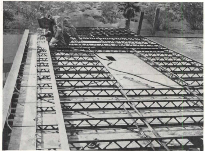
At left: Prefabricated bathroom, showing combined plumbing for bathroom, kitchen, and porch. Steel Craft House by Richard J. Neutra, Architect. Above, upper: Steel skeleton of standard parts, designed to resist lateral forces of earth shock and wind pressure. Richard J. Neutra, Architect. Above, lower: Expanded metal studs cut to length by torch, joined together by welding to produce strong and light building frame.
