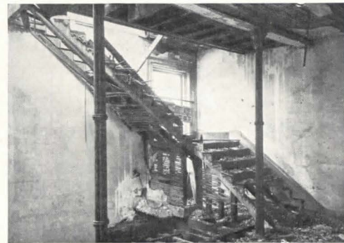
Stairway before restoration
