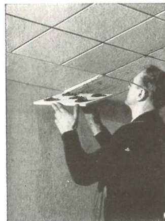
Showing easy application of Tile to ceilings, using adhesive.
