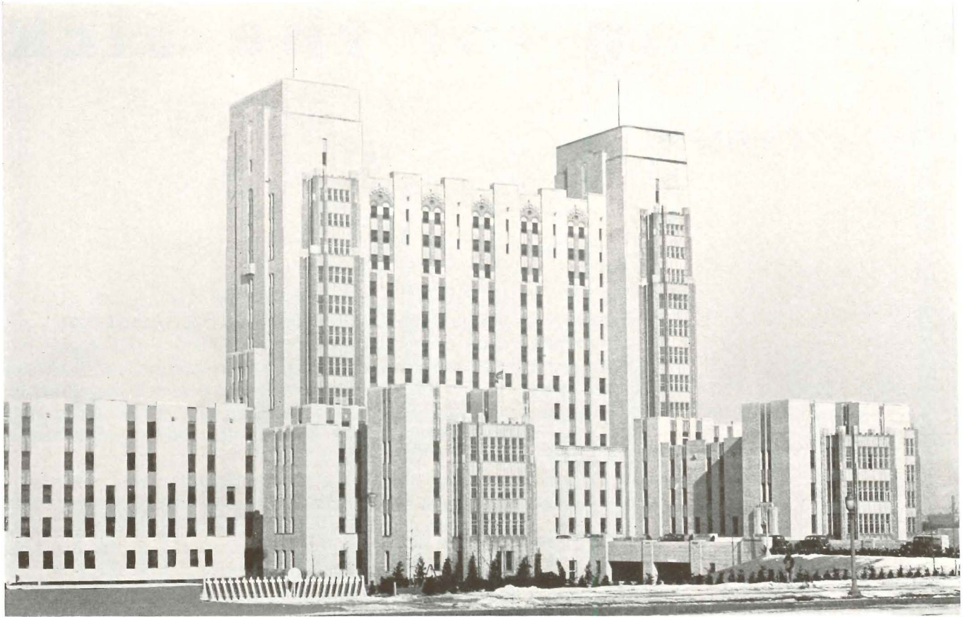
U. S. NAVAL HOSPITAL, PHILADELPHIA, PENNSYLVANIA W. T. KARCHER and LIVINGSTON SMITH, ARCHITECTS
