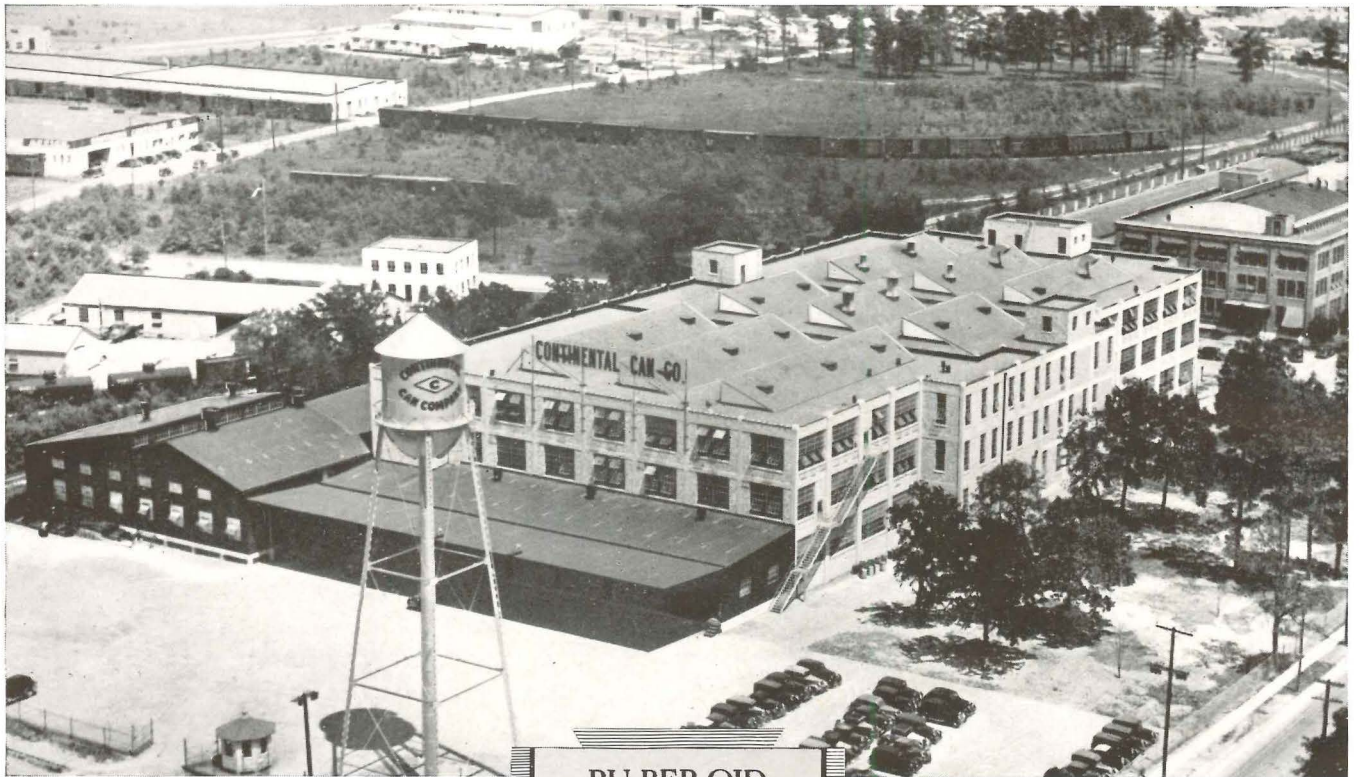
Continental Can Company's Houston, Texas, Manufacturing and Warehouse Building. Protected with 50,000 sq. ft. Ruberoid Built-up Roof.
